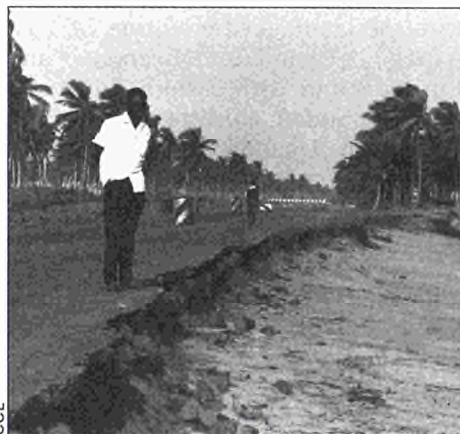
Sea erosion in Togo. Roads are always affected by the elements, but prompt and regular maintenance will keep down costs
