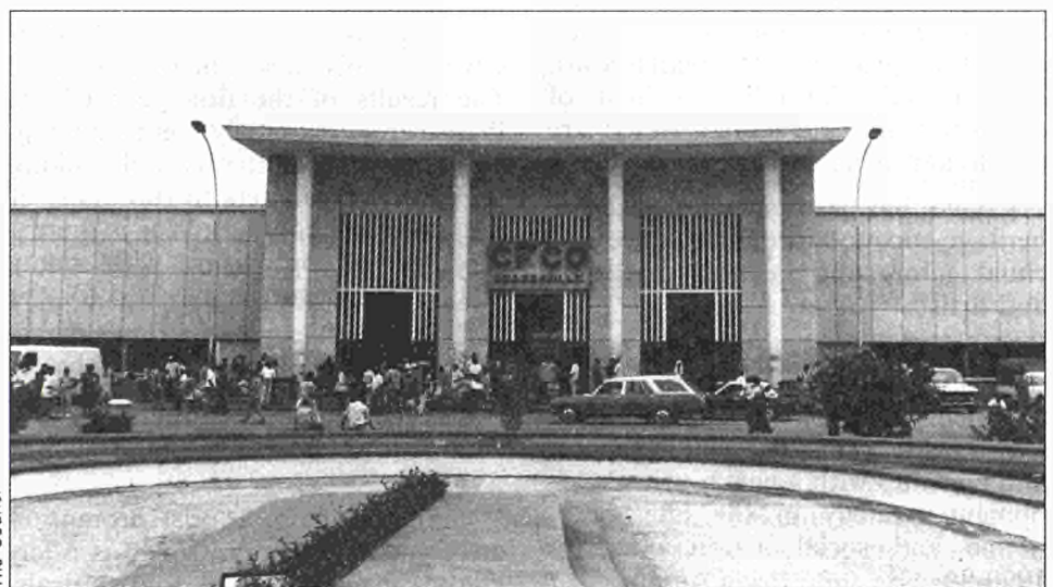
Congo-Océan Railway Station in Brazzaville which has received Community funding for various rehabilitation works
