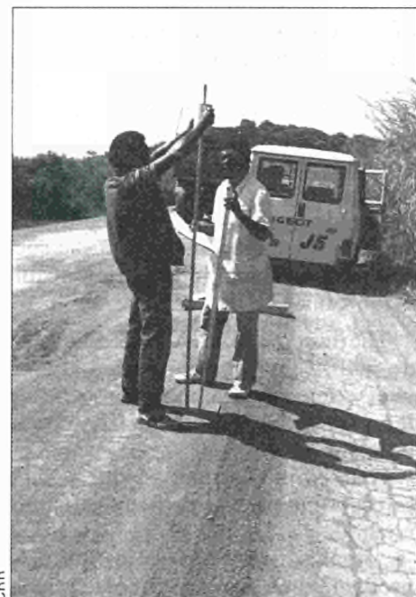
In the field—test drilling
