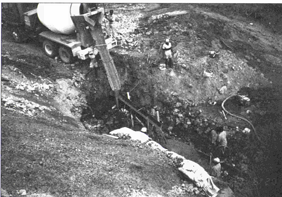
Pouring cement for an underground duct
