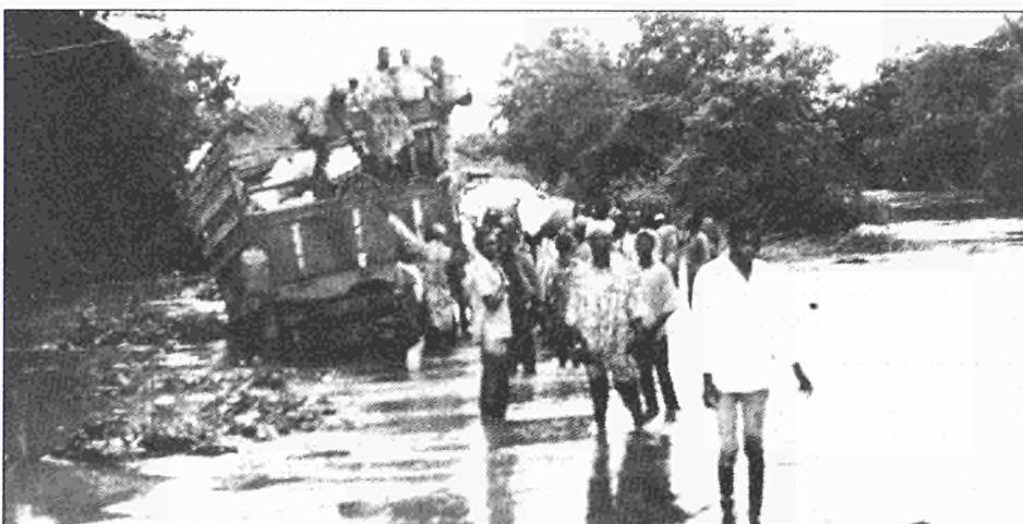
The flood-damaged Iseyin-Saki road
