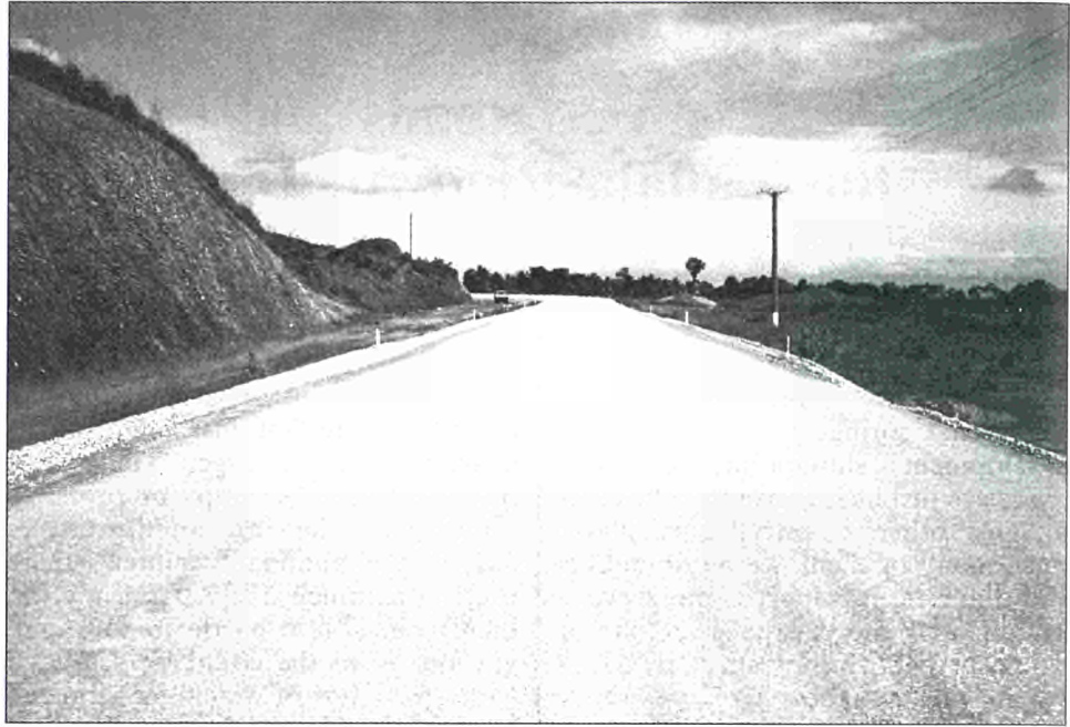
Completion of the base layer at km 34 (towards Rigo)
