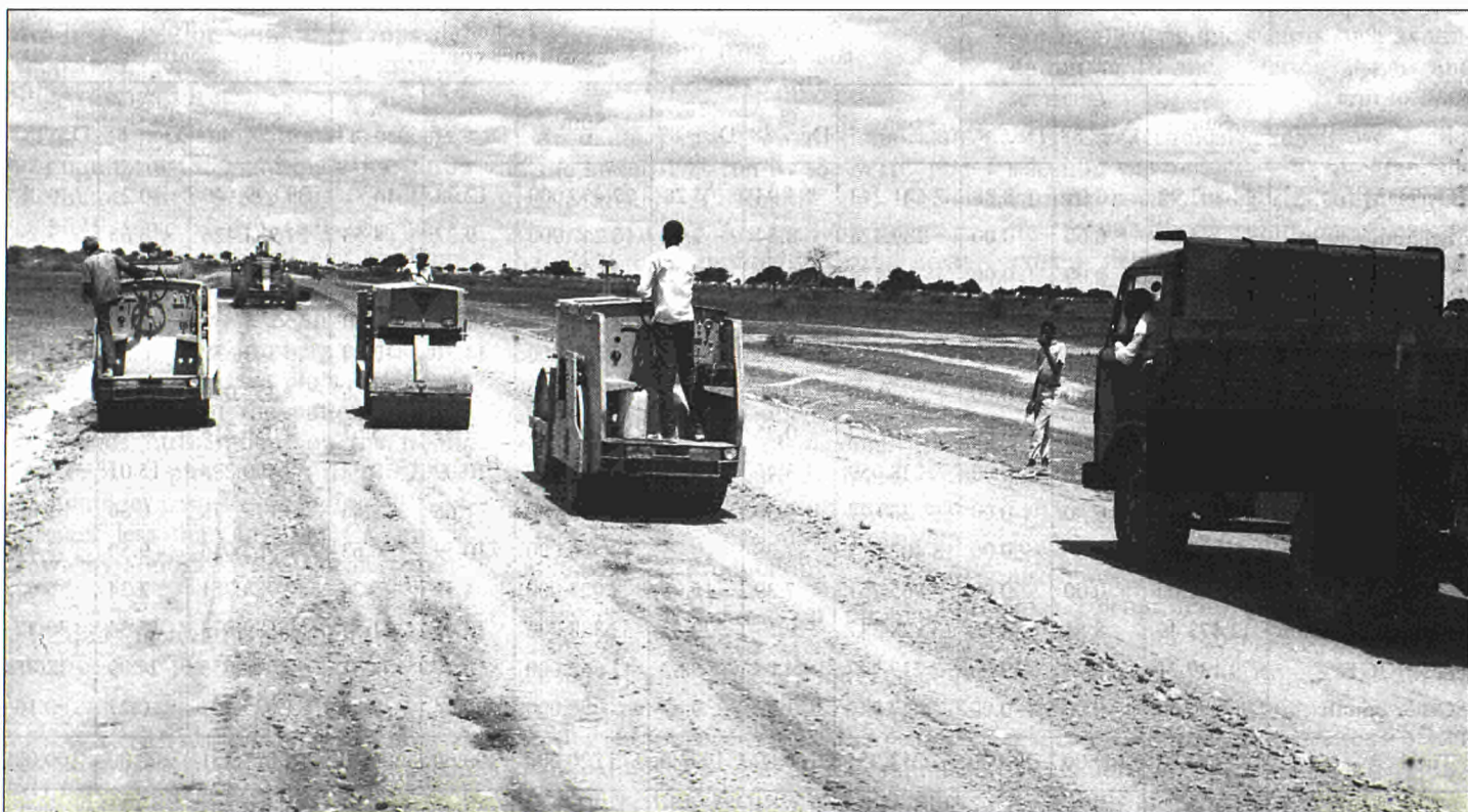
Construction of a road financed by the EDF in Somalia
