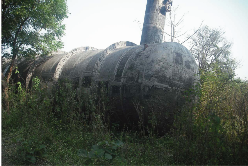
17 FIGURE 1. Tank 610 at the old Union Carbide plant in Bhopal India. Forty tons of toxic methyl 18 isocyanate were released from this tank in the early morning hours of December 3, 1984.
