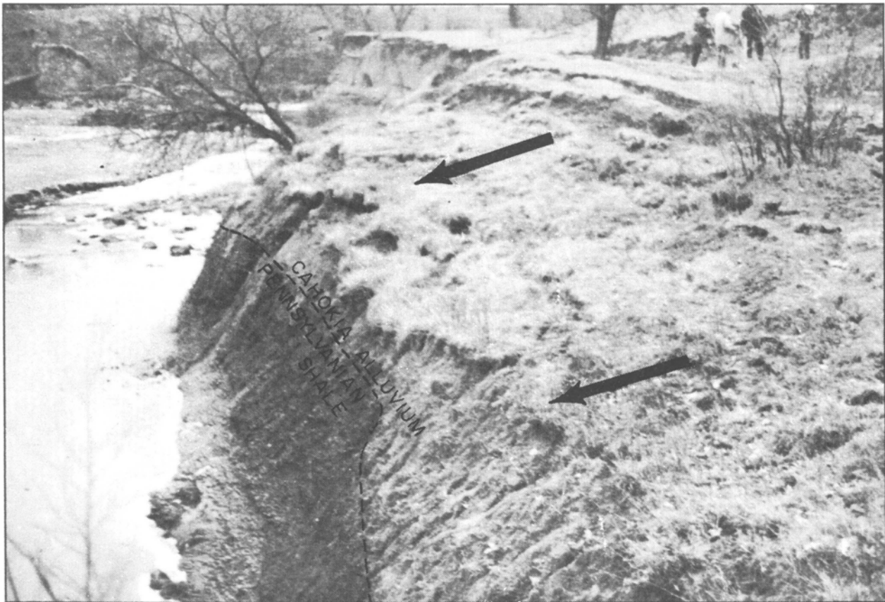
Figure 6 Pennsylvania shale and overlying river alluvium have slumped here along Case Creek in Rock Island County. The entire block (extending from the foreground to the scar beyond the figures in the upper right) has moved toward the creek and has broken into several smaller blocks. Arrows show movement of the block. (Photo: Anderson, 1980)
