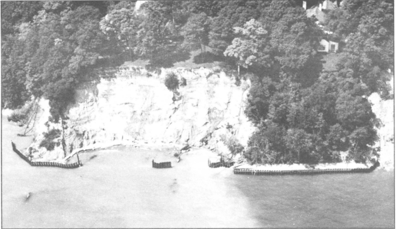
Figure 10 Lake Michigan shore just south of the Lake Bluff Sewage Disposal Plant (1974). The bluff remained vegetated and stable where the bulkhead was maintained. The houses on top of the bluff are less than 50 feet from the bluff edge. In 1975 the bluff toe was protected with riprap and the scarp was filled; the bluff scarp was revegetated and appears stable at the present time (Berg and Collinson, 1976).
