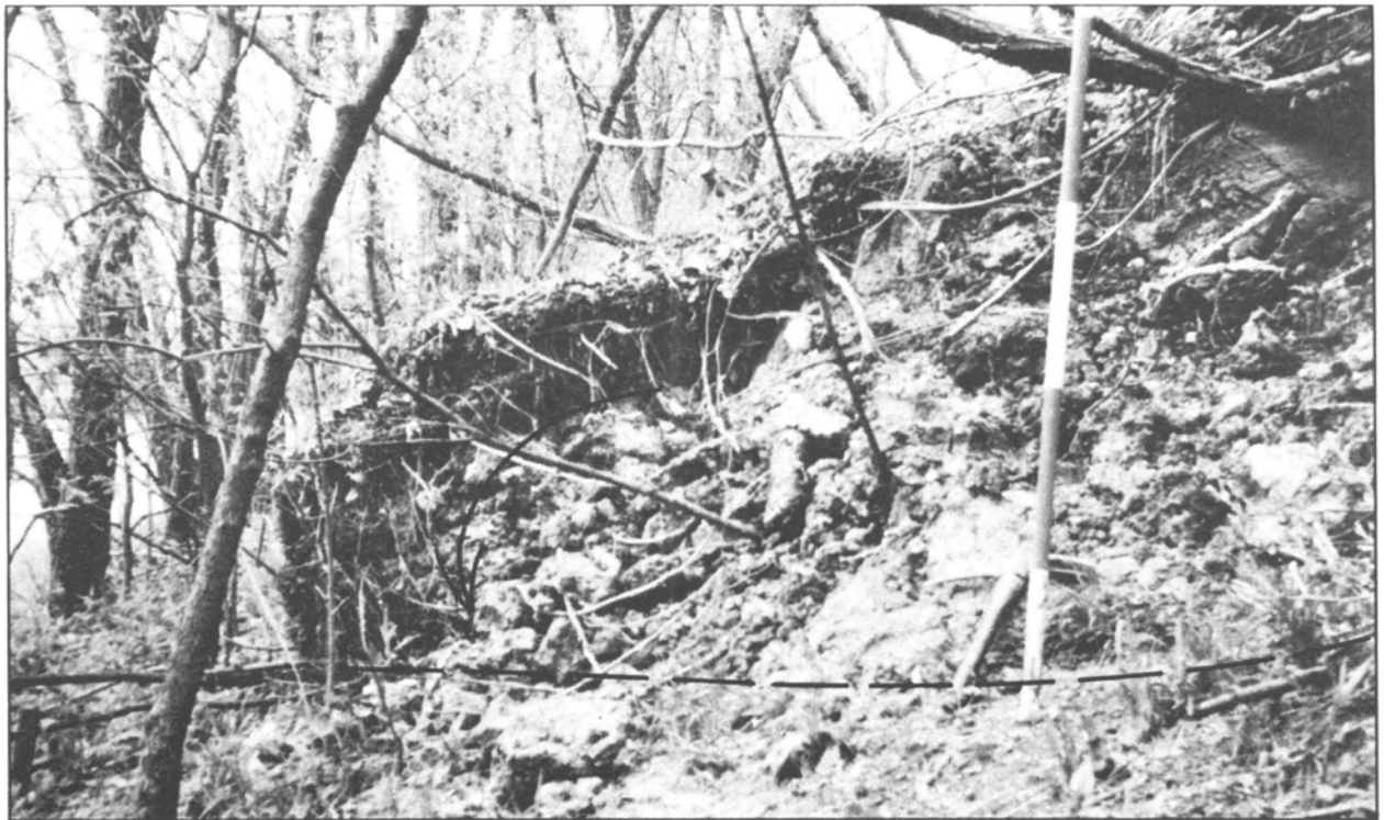
Figure 16 Earth flow occurring as the toe of a large earth slump on bedrock in the bluffs west of the Illinois River. Note the tilted trees on and below the toe. Dashed line shows original ground surface; arrow shows direction of flow. Range pole with 1-foot markings provides a scale.
