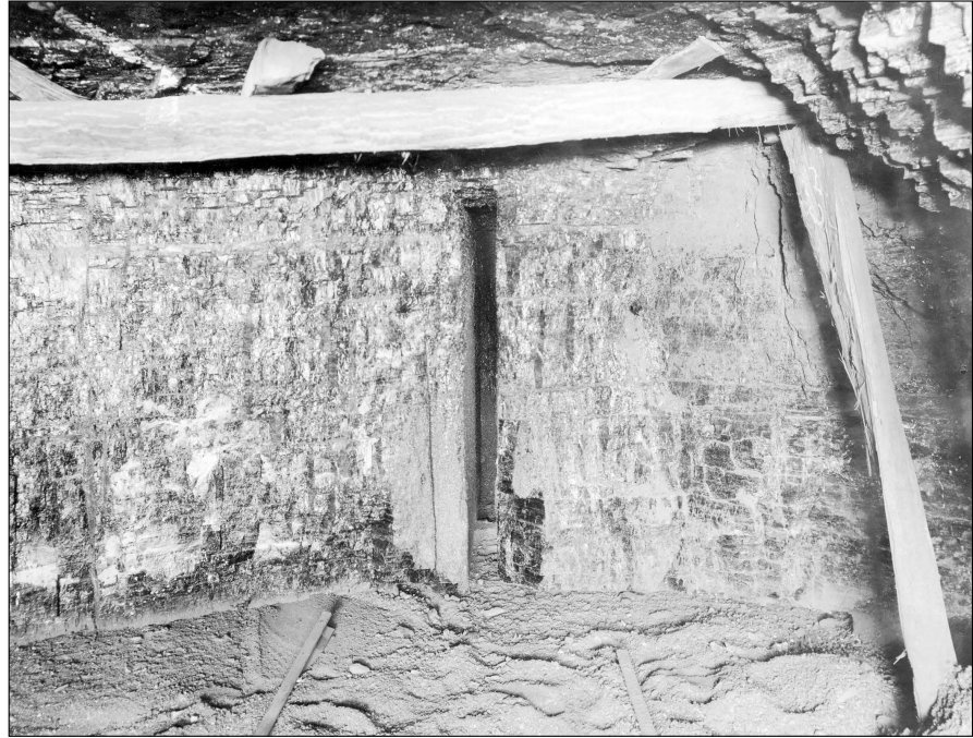
Figure 37 Mine and location unknown. This room has been sheared and undercut and is ready to have the shot holes drilled. Undercutting and shearing are done before drilling to take advantage of any irregularities that result from these processes (Malesky 1973).
