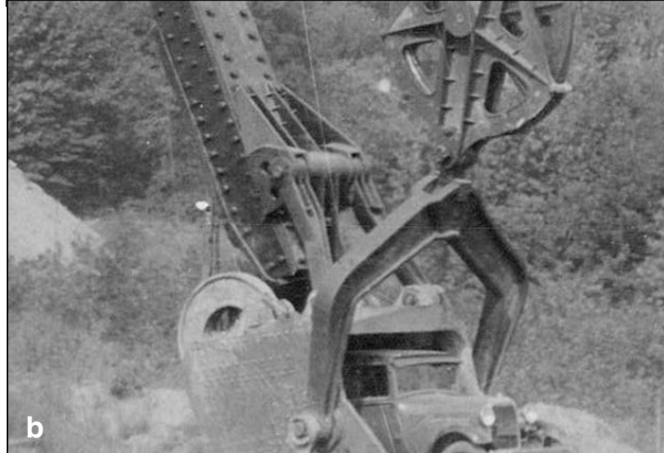
Figure 198 United Electric Company, Fidelity No. 11 Mine, Perry County. (a) The Marion 5600 shovel was another advance in large machines, breaking records when it was introduced in 1929. Note the car parked in the bucket, enlarged in (b), and the rivets on the dipper stick. This was the only Type 5600 built, and it had a 15-cubic yard bucket and weighed 1,550 tons (Historical Construction Equipment Association 2002).
