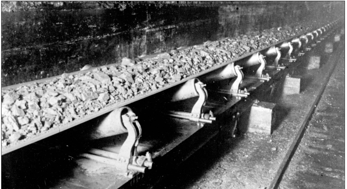
Figure 79 H.C. Frick Coke Company, Bunsen Mine, Vermilion County. This belt conveyor is part of a system 4.5 miles long. It can move 9,000 tons a day, which is typical of a belt this size. The trend in mining has always been to take staged operations and make them continuous. Belt haulage is a prime example of this concept (Ledvina et al. 1992).
