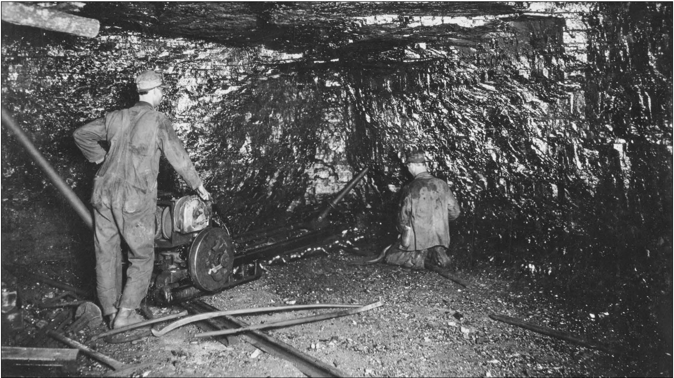
Figure 30 Old Ben Coal Corporation, No. 8 Mine, Franklin County. When the cutting bit of this rail-mounted undercutting machine has dug into the coal the length of the saw portion, it is removed from the coal. Numerous pry bars leverage the machine further along the coal face on the rail.
