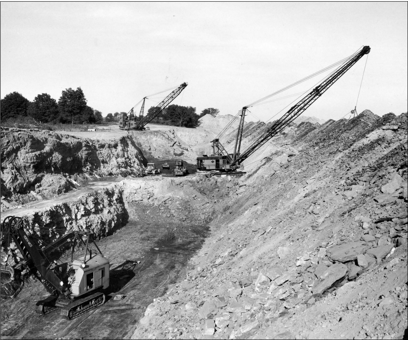
Figure 221 Saxton Coal Company, Newcastle Mine, Saline County. Draglines were used here instead of large stripping shovels to mine two seams in a bench operation. The upper seam is the Dekoven Coal, which is about 20 feet above the Davis Coal in this pit (Ledvina et al. 1992). The dragline in the center of the photograph is resting on the Dekoven Coal, and the shovel in the lower left is working from the top of the Davis Coal.
