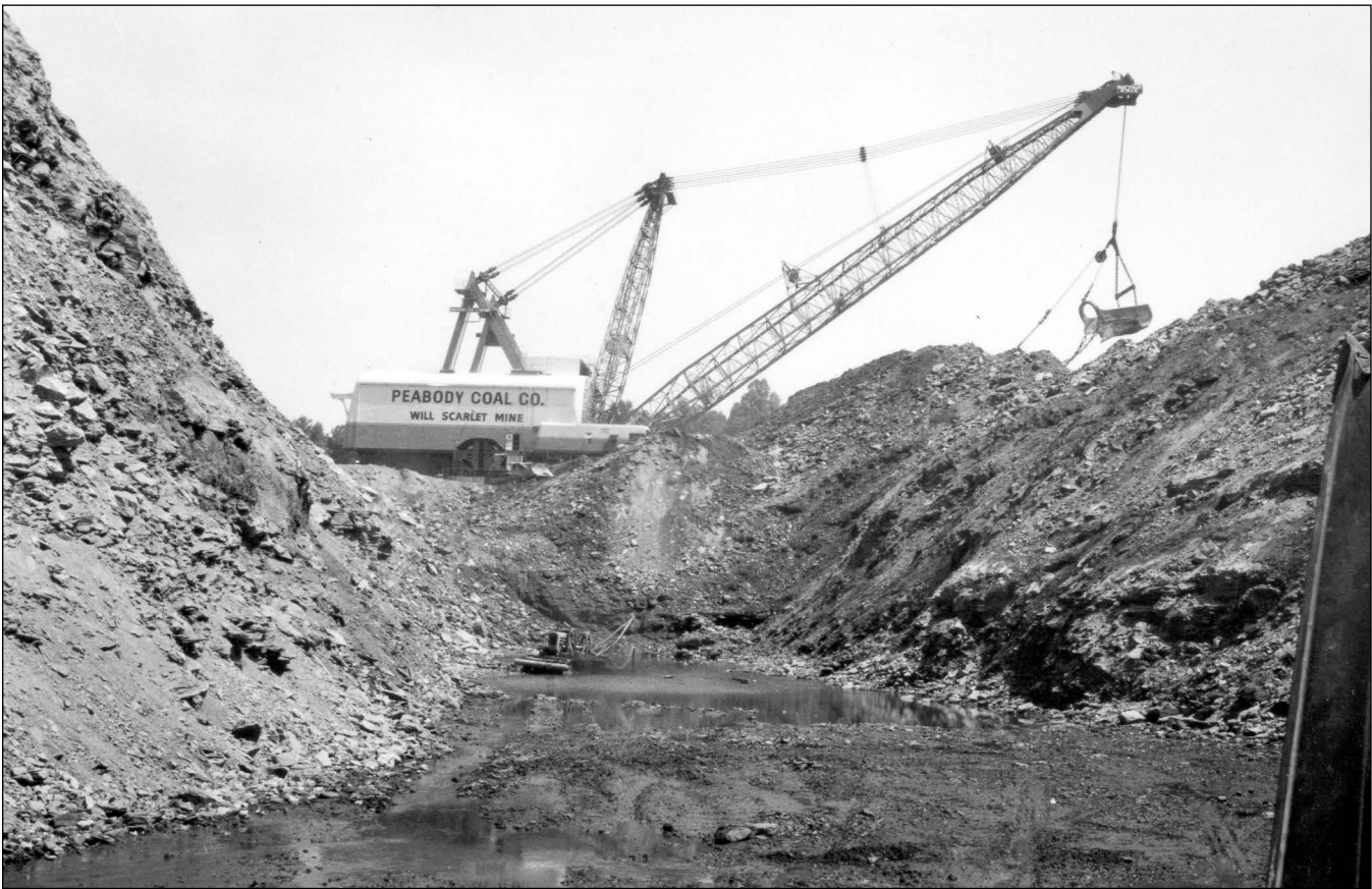
Figure 242 Peabody Coal Company, Will Scarlet Mine, Saline County. This Bucyrus-Erie 1450-W dragline, with an operating weight of 2,916 tons, broke the size record for large draglines when it was introduced in 1963 (Haddock 2001).
