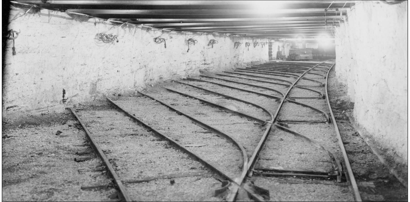
Figure 66 Madison Coal Corporation, No. 12 Mine, Williamson County. An underground motor barn and charging station. This mine probably used battery-powered locomotives for track haulage rather than trolley power (Ledvina et al. 1992).
