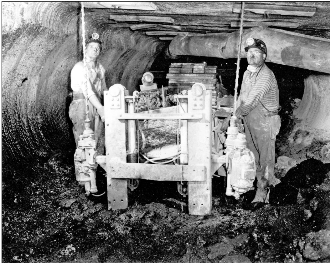
Figure 140 Bell & Zoller Coal Company, No. 3 Mine, near Zeigler, Franklin County. This photograph shows an early dual-boom machine. The operators of this machine work close to unsupported roof. The curved side walls indicate that a boring-type continuous miner excavated this room, and speed was essential to keep up with the advance rate of the mining machine.
