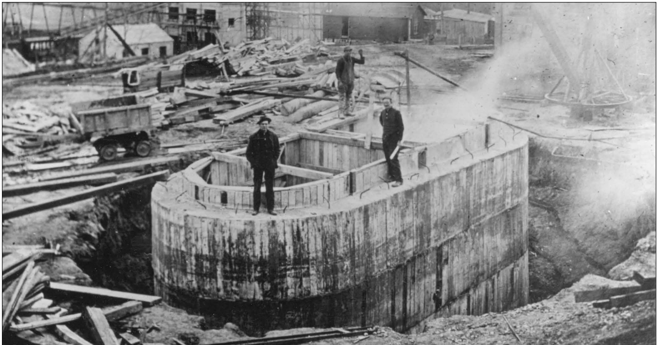
Figure 17 Above: Mine and location unknown. Constructing a shaft was a difficult job without modern equipment. Partitions show separate compartments of the shaft.
