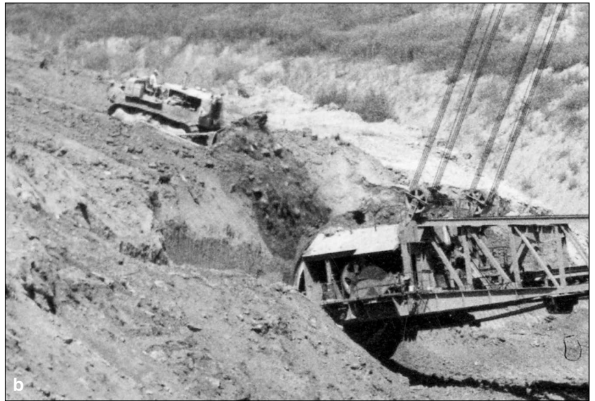
Figure 230 Peabody Coal Company, River King Mine, near Freeburg, St. Clair County. (a) The cutting head of the excavating wheel is shown. The previous cut can be seen above the head, but it is weathered, and the debris has slumped so that the characteristic curved excavation marks are not easily discernible. (b) A bulldozer working in conjunction with the bucket wheel excavator makes an efficient machine even more so.
