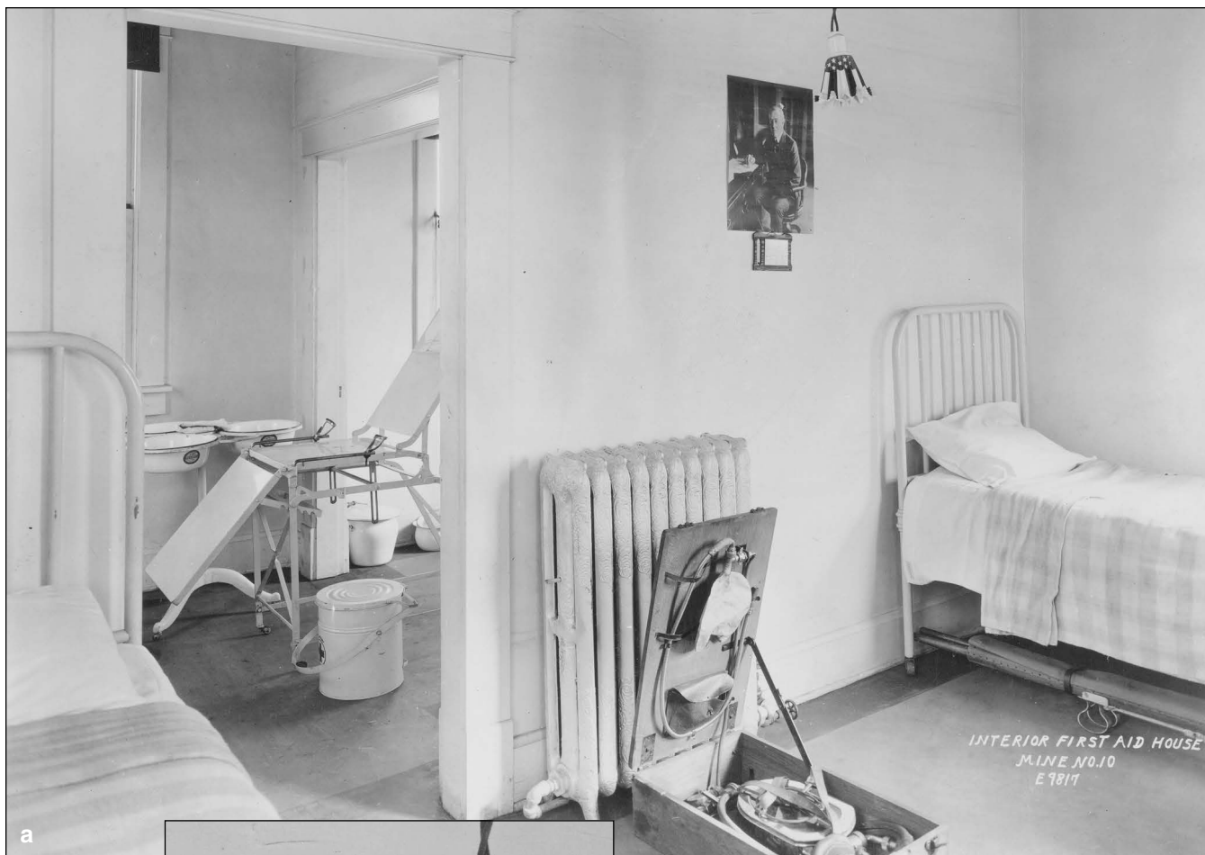
Figure 164 Sahara Coal Company, No. 10 Mine, Saline County. (a) The interior of a mine's first aid house is shown, with an exam chair, hospital beds, and rescue equipment of the times. The box near the radiator can be taken on rescue missions underground and contains breathing apparatus for smoky or gassy conditions. It is clear that this first aid station is a showpiece, a place of pride for the mine to show off. It reflects the utilitarian purpose of the space but is not devoid of ornamentation. The radiator includes decorative elements. The blankets are not plain, but plaids. Money and thought were put into this first aid station to make it a comfortable, home-like place for the injured. (b) The enlargement of a portion of photograph (a) shows the shade for the light that reflects the miners' renowned patriotism with stars and stripes. The photograph is of President Woodrow Wilson.
