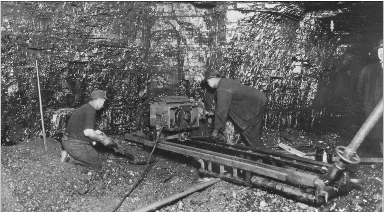
Figure 31 Mine and location unknown. As the coal is undercut by this rail-mounted undercutter, the visible part of the machine is the frame used to guide and drive the bit into the coal.
