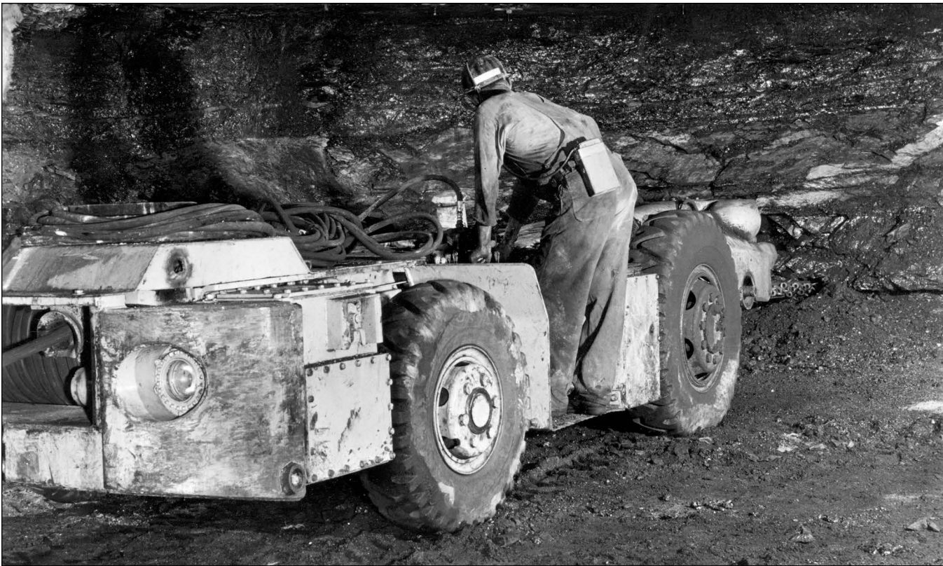
Figure 35 Mine and location unknown. Mounting the undercutter on rubber-tired wheels made a versatile machine that kept the conventional mining technique feasible after the introduction of continuous mining machines.
