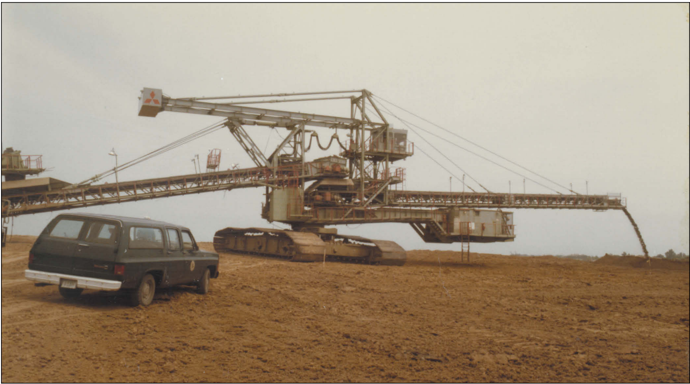
Figure 260 Arch of Illinois, Inc., Captain Mine, near Willisville, Perry County. The Mitsubishi conveyor spreader swung slowly from side to side, depositing the subsoil in an arc onto the rock spoil. Very little grading was required before the topsoil was deposited on top of the subsoil.
