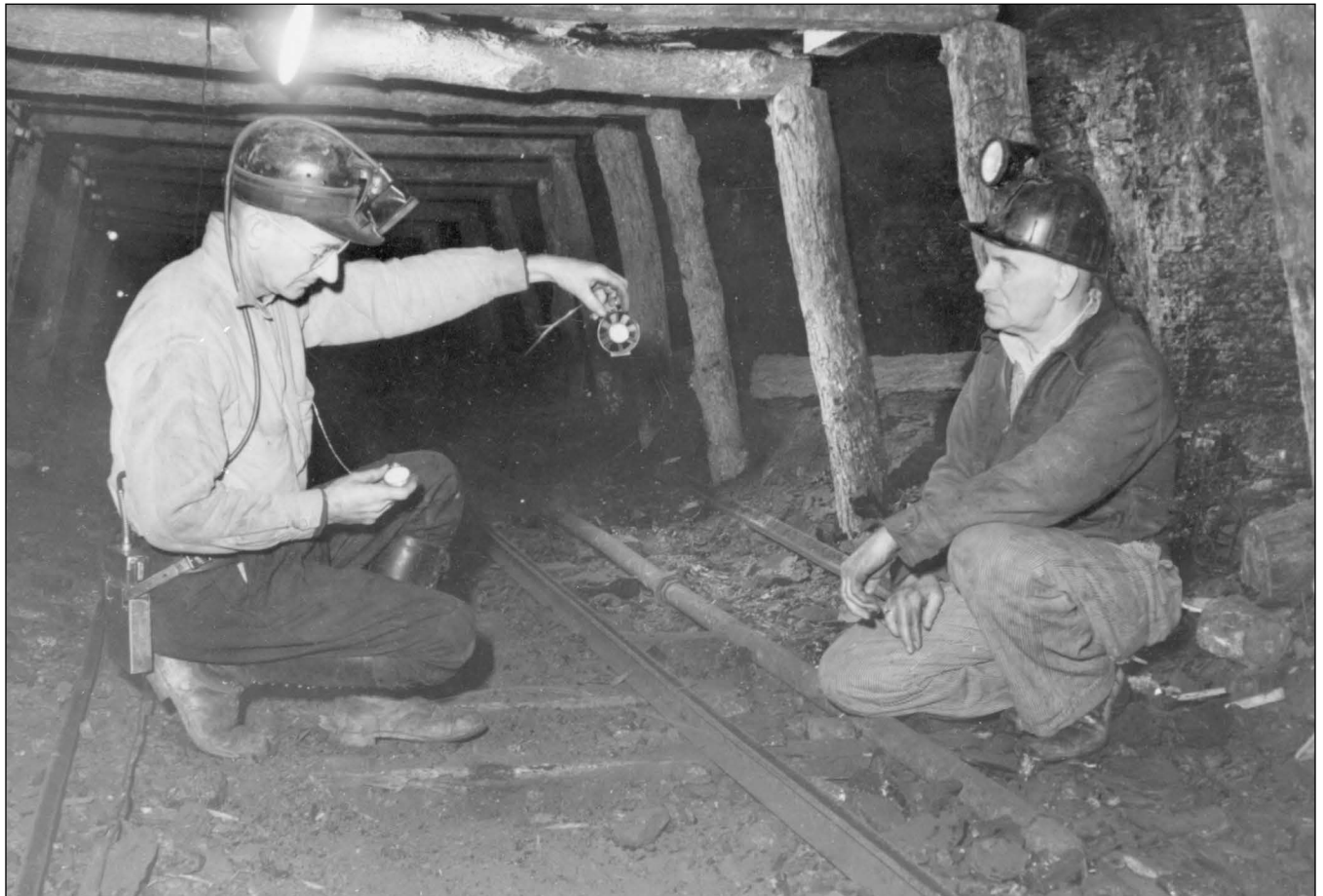
Figure 154 Bell & Zoller Coal Company, mine unknown, near Zeigler, Franklin County. A safety engineer and state mine inspector are shown taking air velocity measurements. The volume of air flow is then calibrated using the cross-sectional area of the entry where the velocity measurement is taken (Jones 1942).
