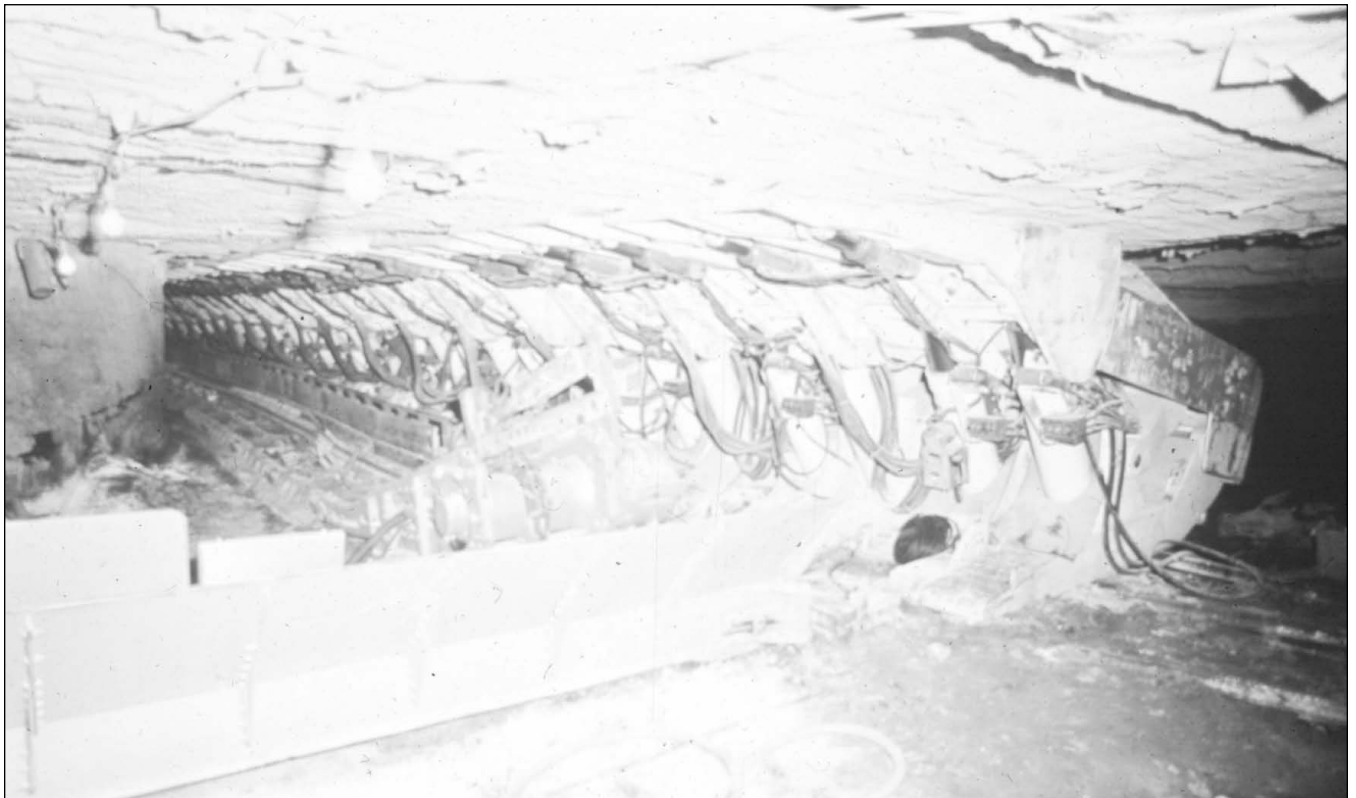
Figure 102 Old Ben Coal Corporation, mine and location unknown. This end of the longwall face shows the side of the shield supports.
