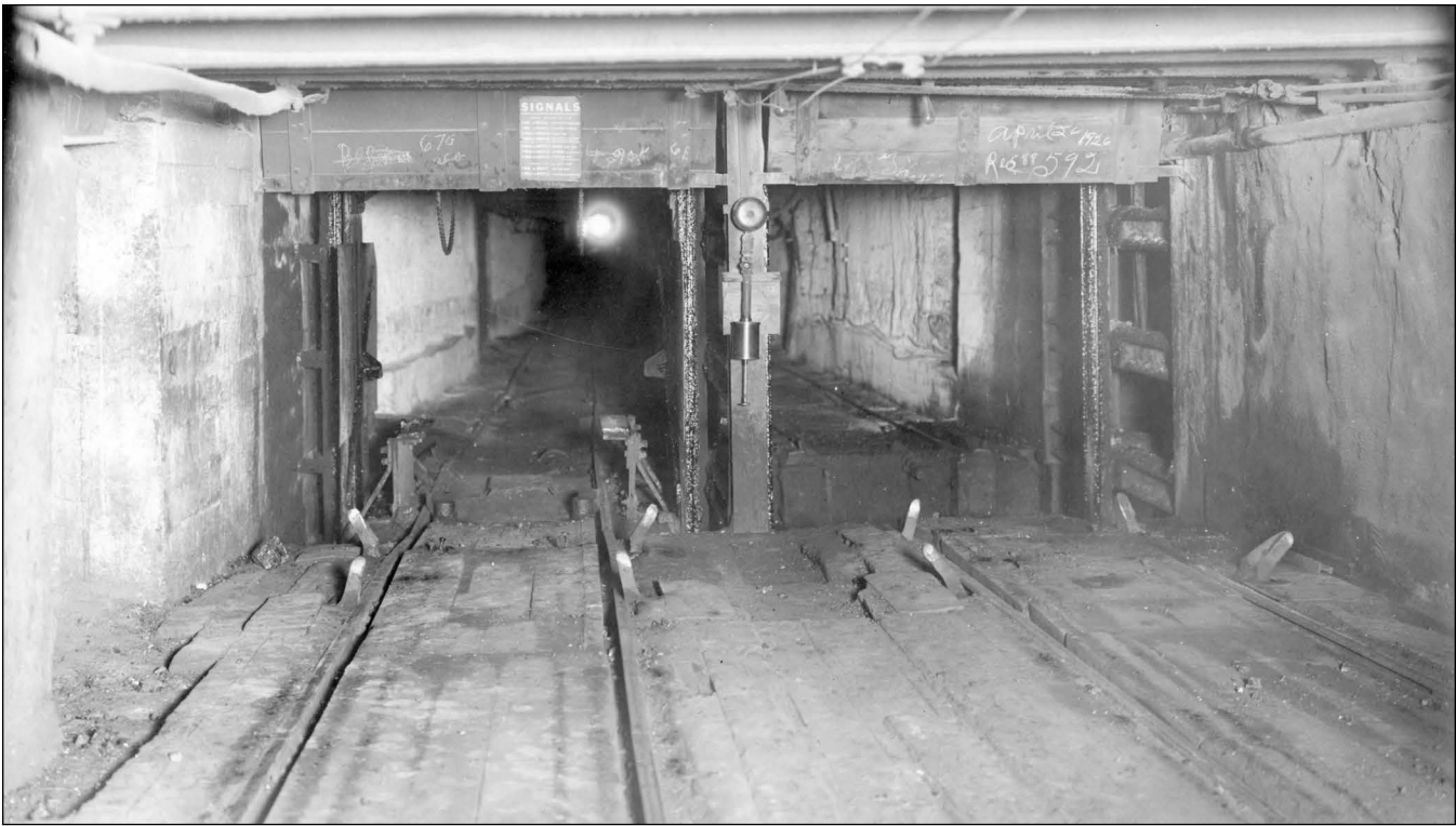
Figure 111 Madison Coal Corporation, No. 12 Mine, near Cambria, Williamson County. The shaft bottom showing automatic caging equipment. The levers near the track block the wheels of the next car once one is on the hoisting platform. After the first car is past the second set of levers, the hoisting platform is released and raised up for dumping.
