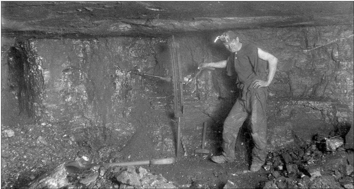
Figure 38 Mine and location unknown, probably Vermilion County. Drilling shot holes with a hand-powered auger-type drill. This photograph was probably taken between 1900 and 1915.
