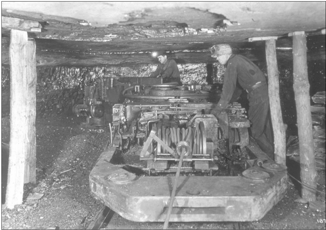
Figure 34 Mine and location unknown. This undercutting machine was an advance on previous versions. Although this undercutter required rails, the head rotated so that it could undercut coal to the left, in front, and then on the right side of the machine without laying additional track. Track-mounted machines were made obsolete by machines mounted on rubber tires in 1946 (Morrow 1962).
