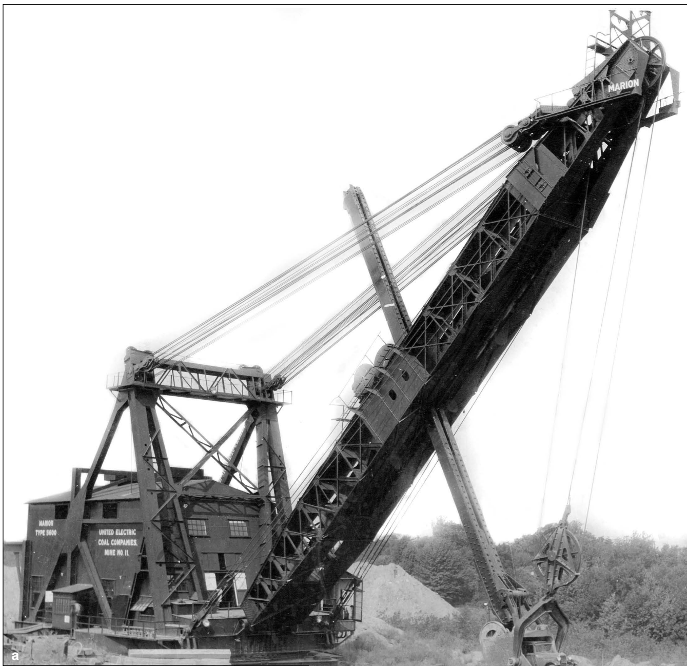
Figure 198 United Electric Company, Fidelity No. 11 Mine, Perry County. (a) The Marion 5600 shovel was another advance in large machines, breaking records when it was introduced in 1929. Note the car parked in the bucket, enlarged in (b), and the rivets on the dipper stick. This was the only Type 5600 built, and it had a 15-cubic yard bucket and weighed 1,550 tons (Historical Construction Equipment Association 2002).
