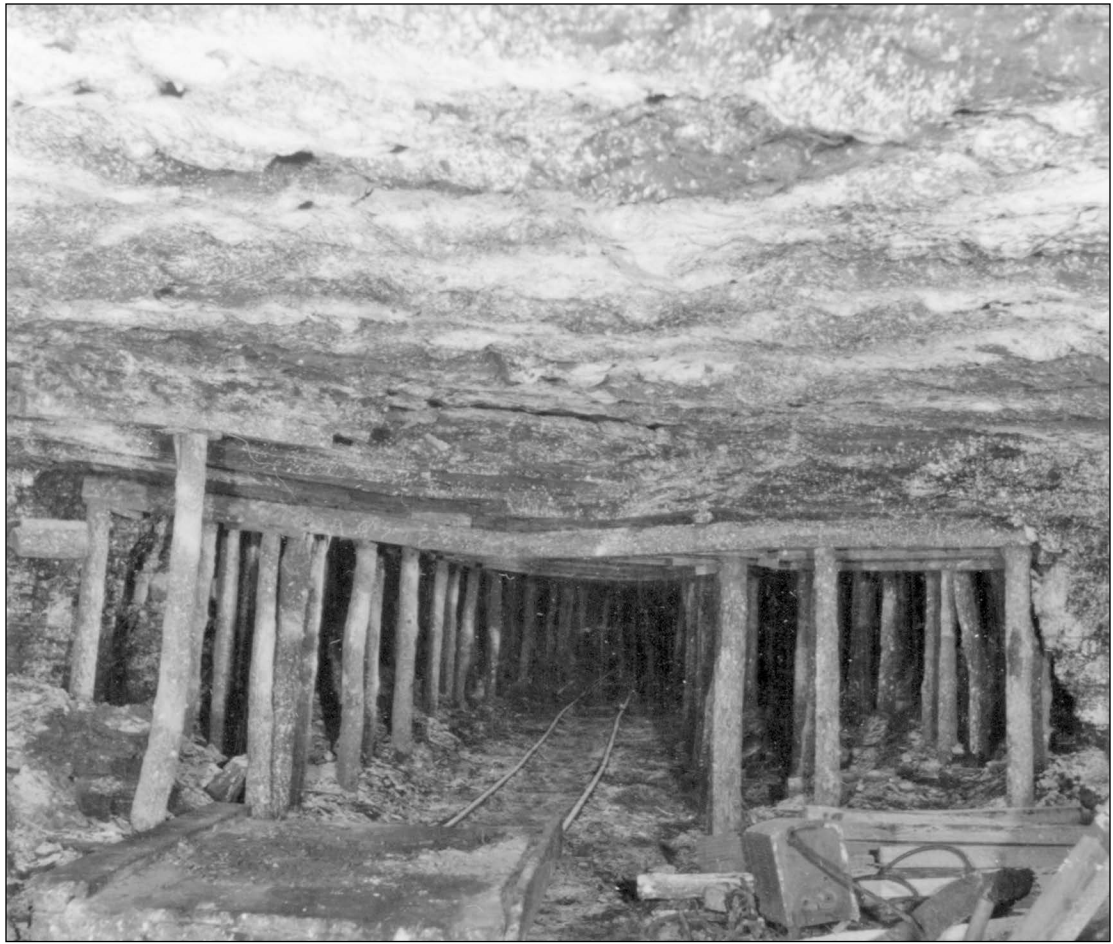
Figure 152 Bluff Coal Company, St. Clair County. The roof in this area is 3 feet of black shale that required heavy timbering, but generally came down anyway. Above the shale, in the photograph foreground, the lower surface of the limestone was relatively smooth.
