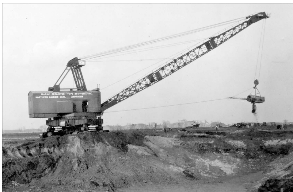
Figure 196 Northern Illinois Coal Corporation, Northern Mine, Will County. The Marion 5480E electric shovel was crawler-mounted and had a 12-cubic yard bucket (Hollingsworth 1963) and weighed 975 tons (Historical Construction Equipment Association 2002). This machine also featured a three-part hoist, inside dipper stick, and rack and pinion crowd. At about this time, Bucyrus constructed Model 750-B, which had twin hoist ropes on the dipper. This model helped eliminate an old shovel problem, when one side of a dipper caught on a rock or hard spot and twisted the front end, cracking the dipper stick or warping the boom (Hollingsworth 1963). The rails extending from the rear portion of the housing are for an internal crane that aided maintenance and repairs. Doors in the back could be opened to bring in equipment (Historical Construction Equipment Association 2002).
