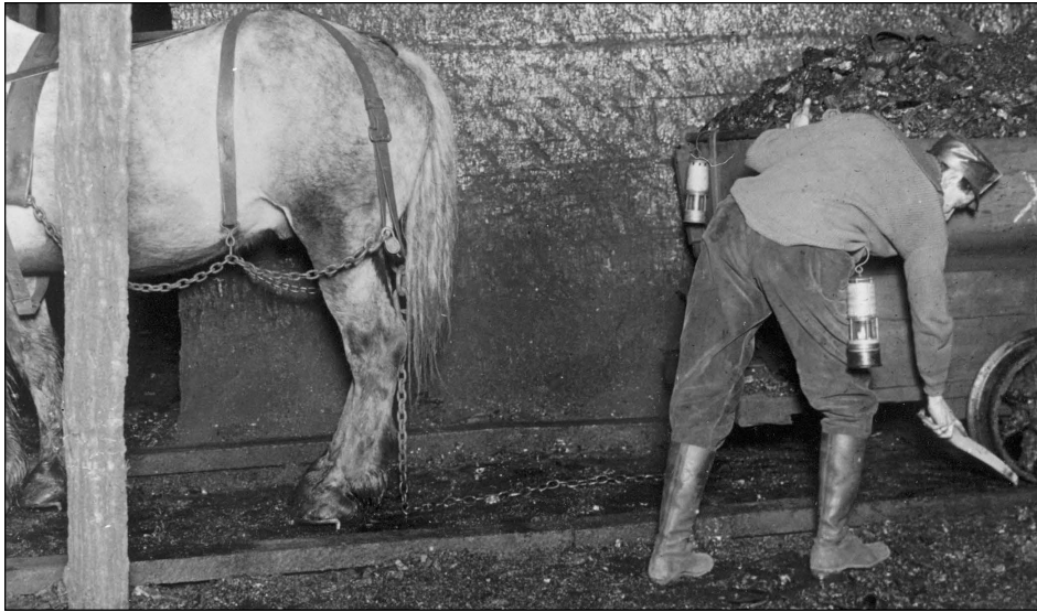
Figure 63 Mine and location unknown. This driver is placing a wedge to prevent the loaded car on the track from rolling. In many mechanized mines, horses and mules were used to haul the coal cars to a main haulage route to make a train, or "trip," of loaded cars to be taken to the hoist shaft (Ledvina et al. 1992).
