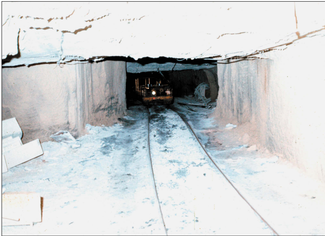
Figure 101 Old Ben Coal Corporation, mine and location unknown. Longwall mining units require access to the coal that must be developed using continuous mining machines. These rock-dusted entries are also used for haulage and ventilation.
