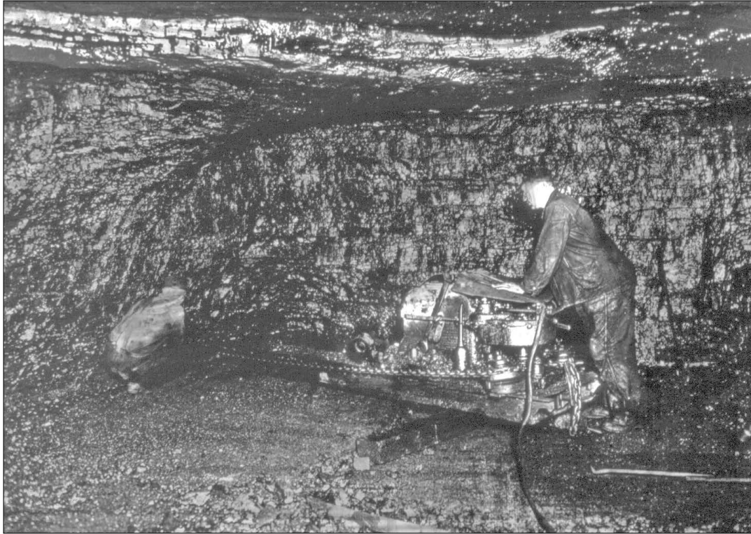
Figure 28 Mine and location unknown. This undercutter uses a regular chain to work the material under the coal loose. The back of the machine is tilted upward on a block of wood. The photograph is too dark to see the blade, but the machine is similar to the 1899 Sullivan CE shortwall cutter (Morrow 1962).
