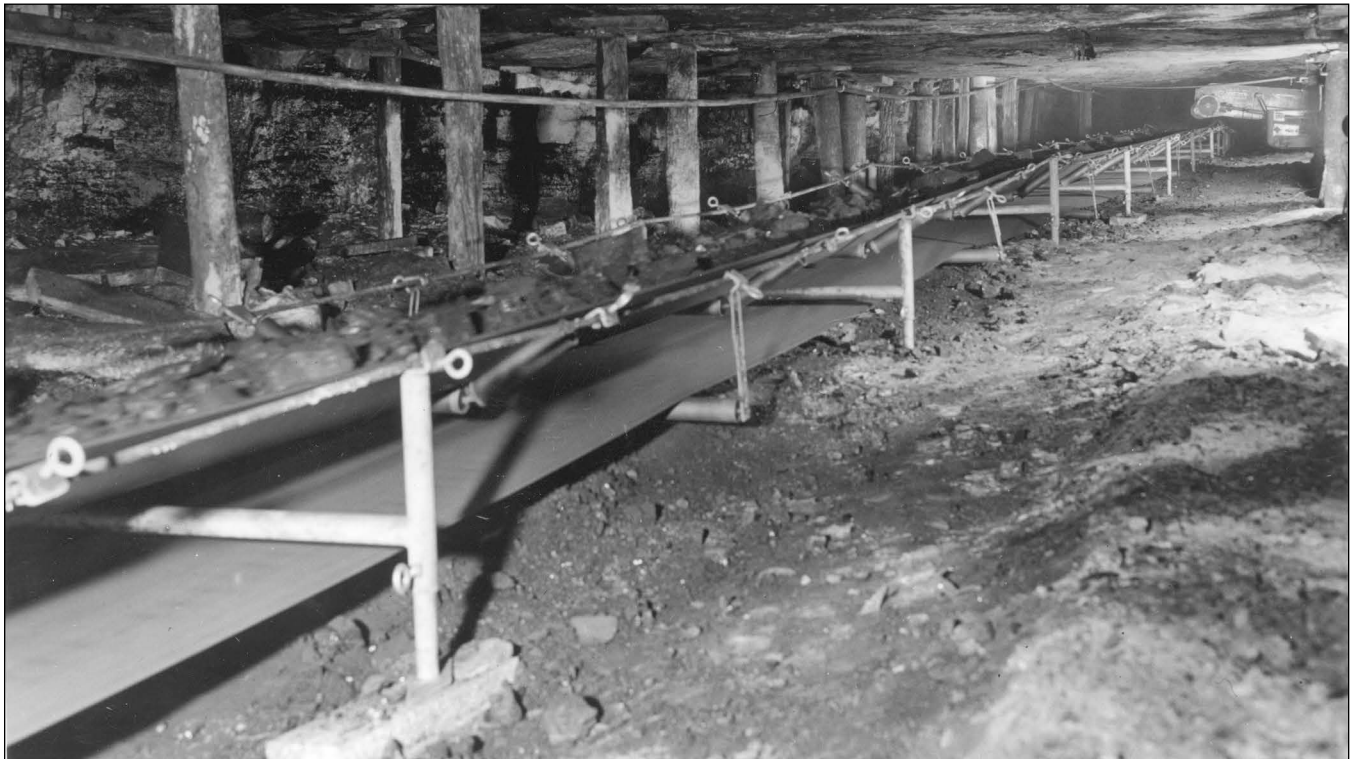
Figure 106 Mine and location unknown. Conveyor systems such as this one could be miles long and led directly to the main shaft or up the slope to the preparation plant. Later systems were developed that were mobile and could be attached directly to the continuous miner (Ledvina et al. 1992).
