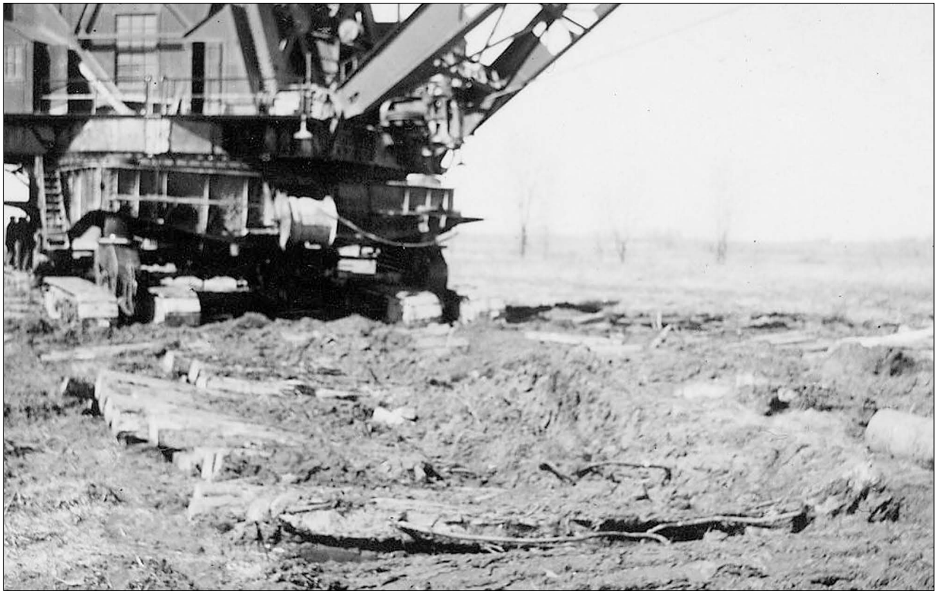
Figure 205 Northern Illinois Coal Corporation, Northern Mine, Will County. The condition of the timbers after the dragline has passed over them shows that the weight is still enough to crush them and compress the soil under the machine.
