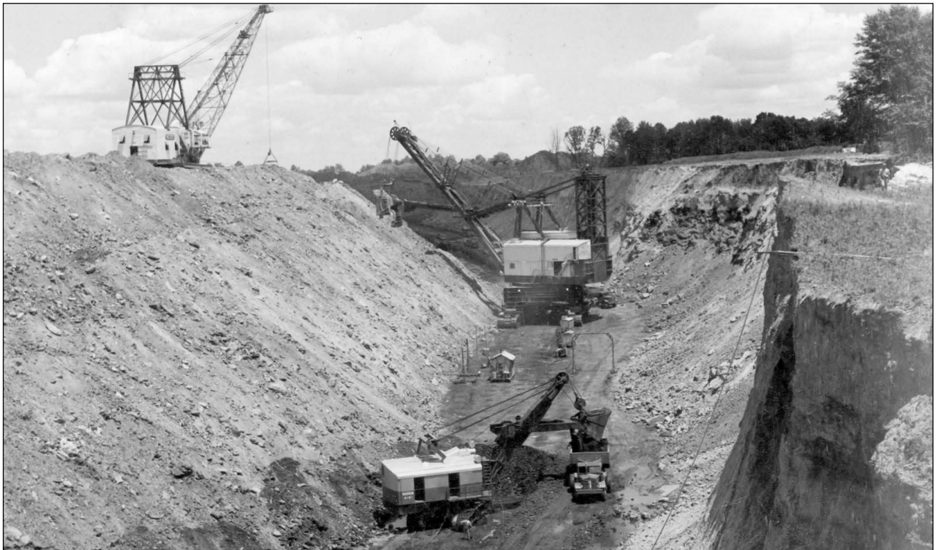
Figure 223 Mine unknown, perhaps Harmattan Mine, Vermilion County. This photograph shows the typical configuration of surface mines in the latter half of the twentieth century. The dragline on the spoil pile rehandled the spoil so that the piles did not slide back into the pit as the shovel added material. A bulldozer cleaned the top of the coal and sometimes aided the loading shovel.
