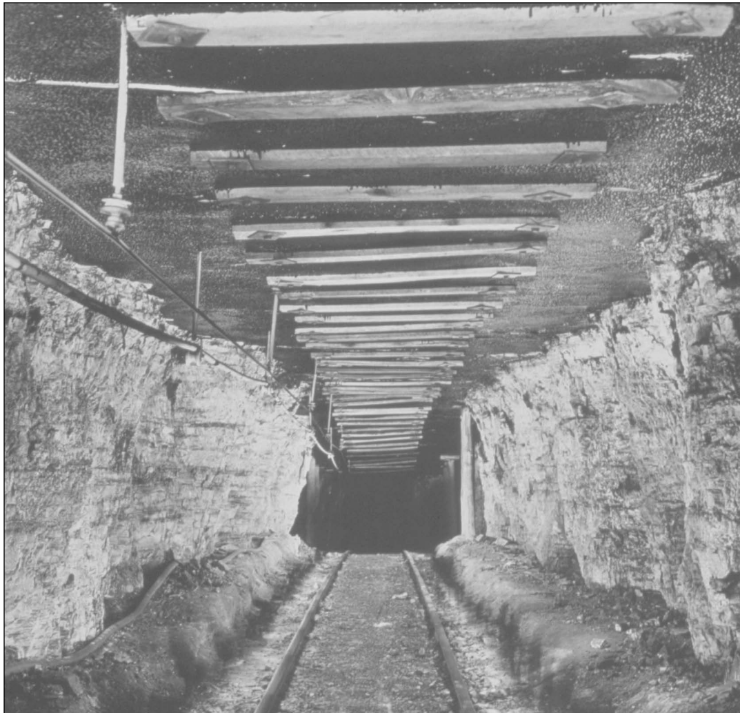
Figure 150 Mine and location unknown. This sloping entry used bolted planks to support the roof above a haulage route.
