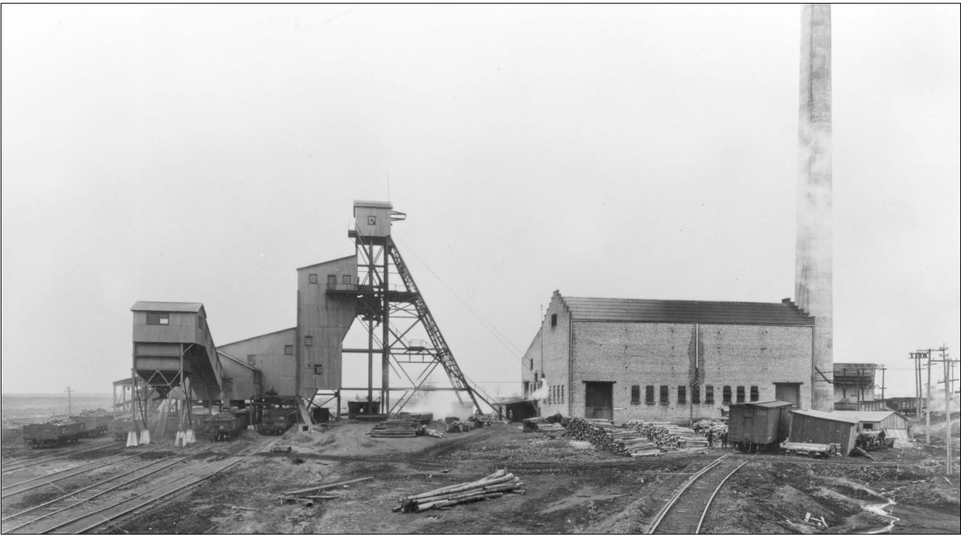
Figure 5 Old Ben Coal Corporation, No. 11 (or New North) Mine, Franklin County. Mines often constructed railroad spurs that stored the cars for hauling their coal to market. The large A-frame structure (head frame) in the center was the location of the hoist shaft, and the building to the left was the sorting shed and tippel. A pile of timbers to prop the mine roof can be seen in front of the building on the right, which probably contained mine offices, hoisting equipment, and machine shops. This mine was the site of an explosion on Thanksgiving Day in 1917.
