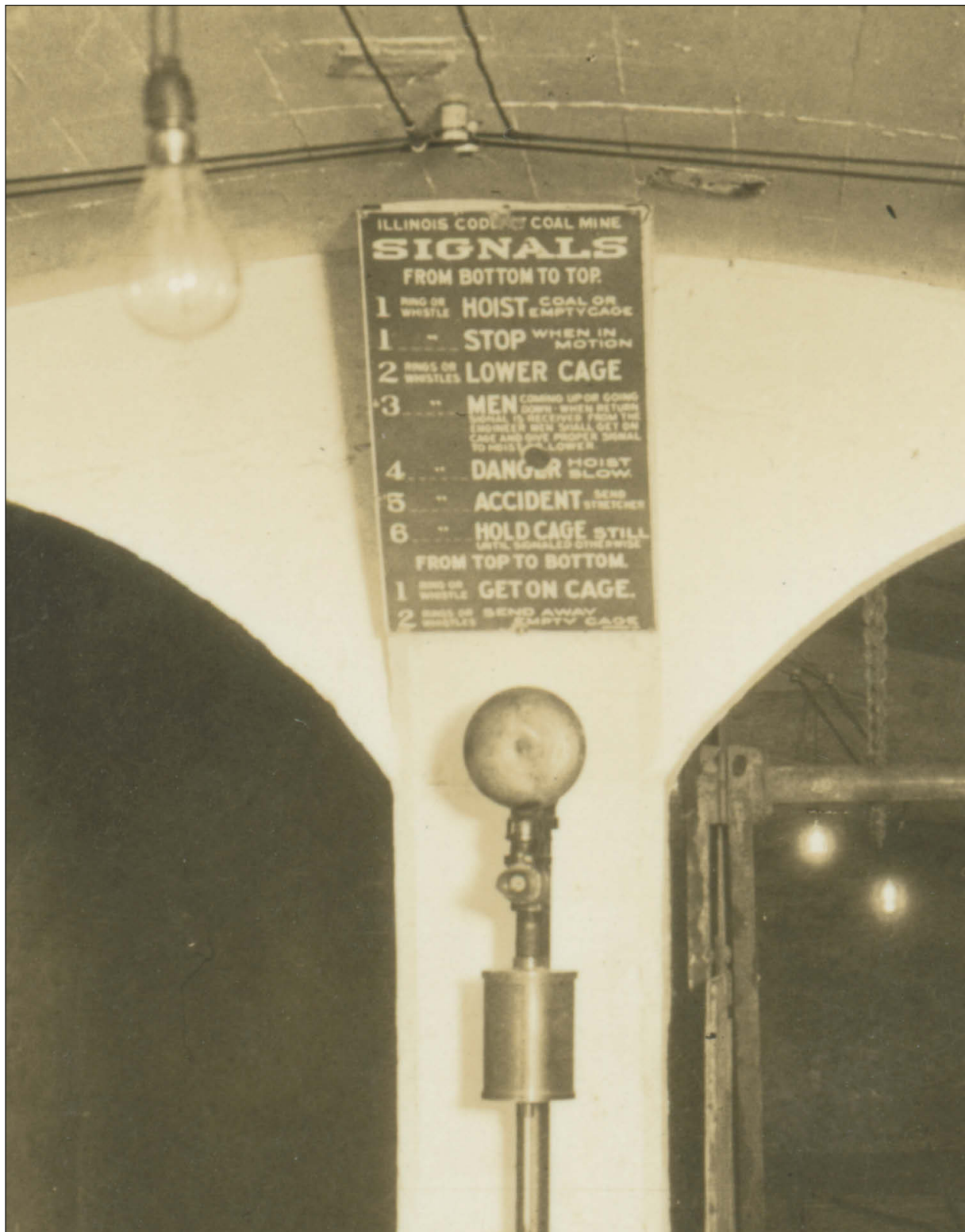
Figure 115 Big Creek Coals, Inc., No. 4 Mine, Saline County. Detail from Figure 113 on the previous page. The signal bell and codes for the bell are shown. Only the most succinct of messages could be given. The hoisting engineer on the surface would signal that the cage was about to be lowered, or the cagers at the shaft bottom could signal to the hoisting engineer to raise the cage. Later communication developments did add a margin of safety; several deaths resulted from confusion about these hoisting signals.
