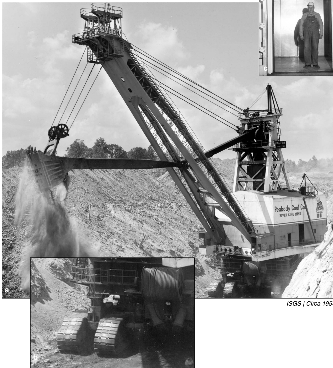
Figure 224 Peabody Coal Company, River King Mine, near Freeburg, St. Clair County. This Marion 5760 electric stripping shovel, “Big Paul, the King of Spades,” built in 1958, was the first of three similar giant excavators to be owned or operated by Peabody Coal Company. The last, a Bucyrus-Erie 3850-B, with a 115-cubic yard bucket on a 210-foot boom, was taken out of service during the summer of 1992 when River King’s reserves were depleted. Big Paul’s 140-foot boom could load 100 tons of overburden and move it one city block away (Sheley 1935) onto a 100-foot high spoil heap. For support and mobility, this machine used four sets of dual crawlers that were connected to the frame with massive hydraulic jacks to make certain the load was dispersed equally in a horizontal direction. The enlarged portion (b) shows the hydraulic jacks and the crawlers that supported Big Paul’s 2,750-ton weight. The operator’s elevator (c) was standard on large shovels after 1956. First introduced on “The Mountaineer,” Marion’s first 5760, the elevator was in the center pin and allowed access to the moving upper deck from the stationary lower deck while the shovel was working (Haddock 2001).
