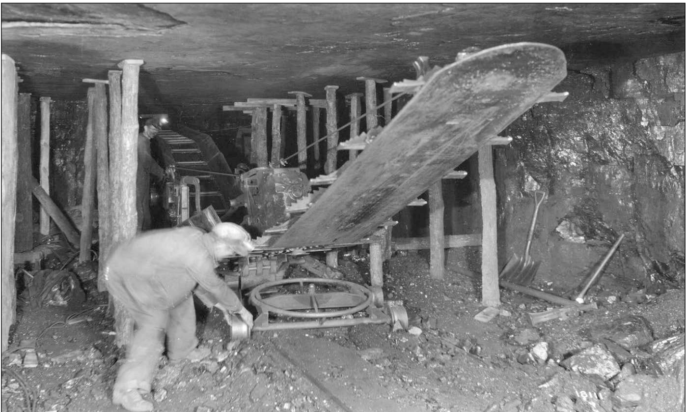
Figure 52 Peabody Coal Company, mine and location unknown. This duckbill loader is attached to an early conveyor.
