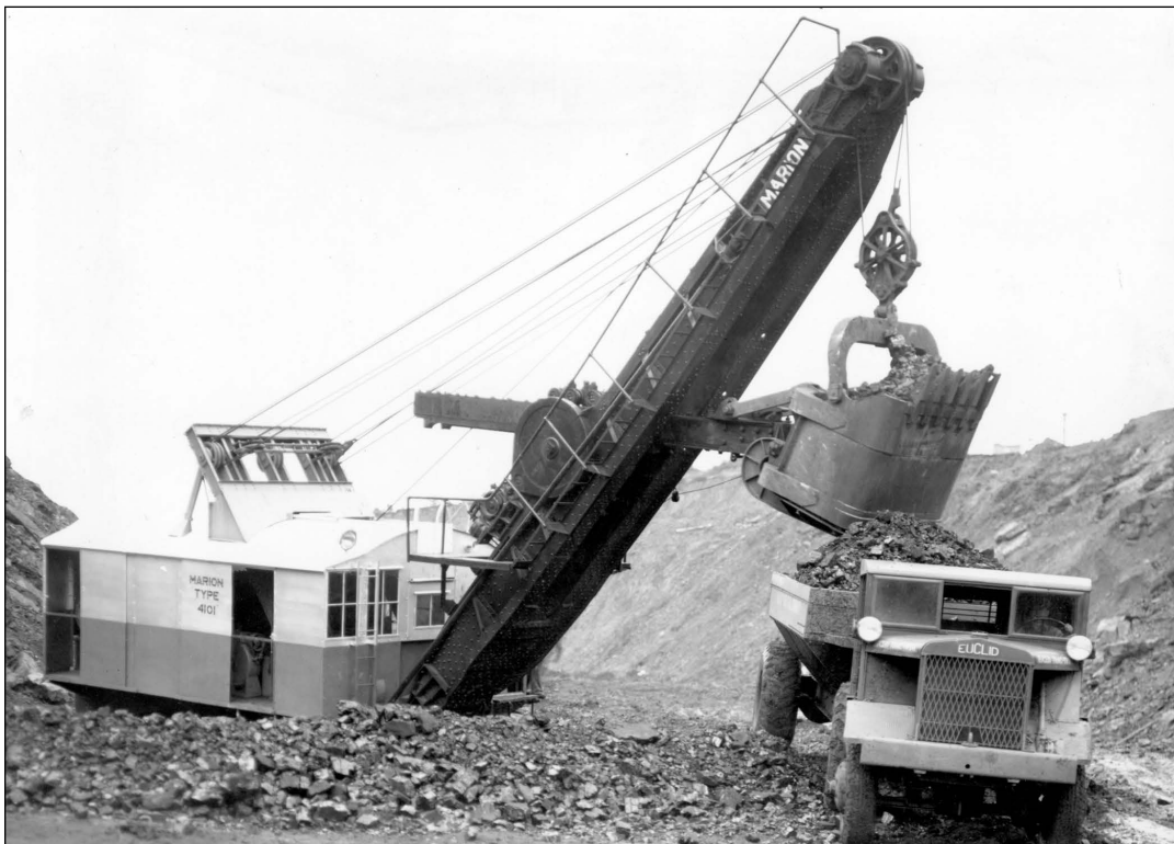
Figure 202 Little Sister Coal Company, Little Sister Mine, near St. David, Fulton County. Bucyrus-Erie 5-cubic yard 85-B loading shovel (Williamson and Myers 1955) and Caterpillar Diesel bulldozer with Bucyrus-Erie blade working in tandem.
