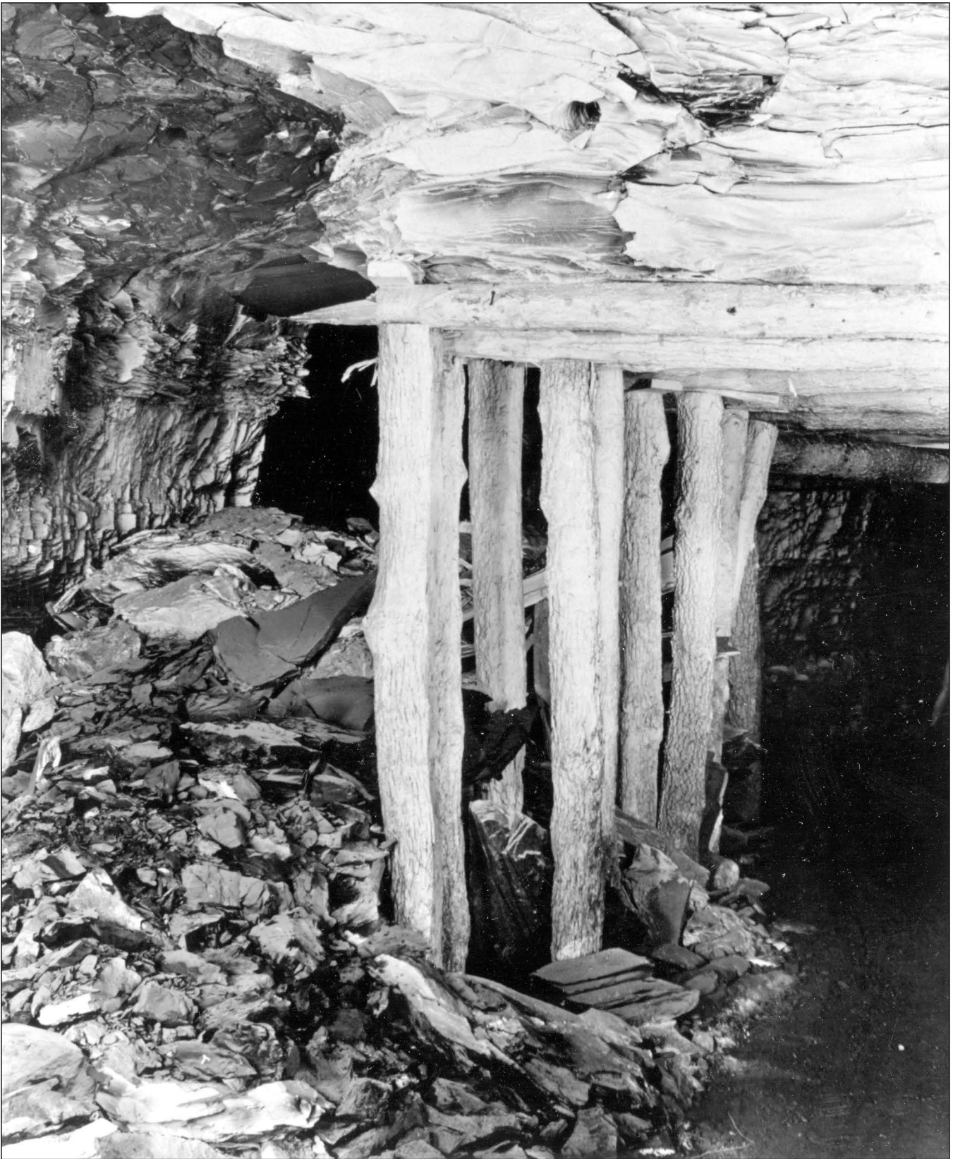
Figure 132 Consolidated Coal Company, No. 7 Mine, near Staunton, Macoupin County. This roof fall is probably a gray shale. Note the closely spaced timbering used to support the roof over the haulage route (Ledvina 1992).
