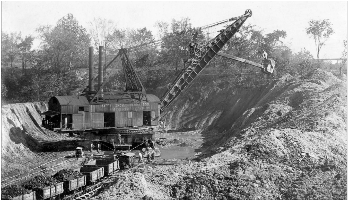
Figure 181 Mission Mining Company, west of Danville, Vermillion County. This Marion 300 steam shovel had a 6-cubic yard bucket and weighed 350 tons (Historical Construction Equipment Association 2002).
