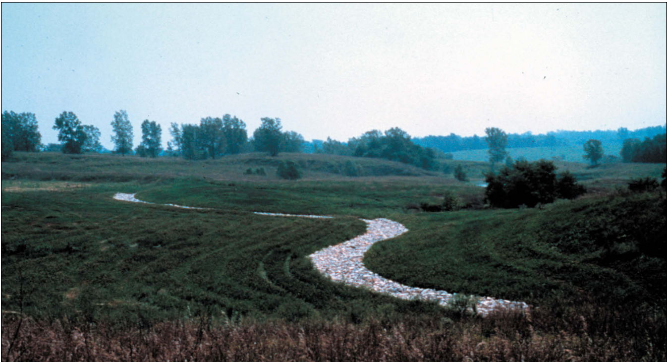
Figure 282 Amax Coal Company, Sunspot Mine, Fulton County. Top soil and subsoil are replaced in their natural order in reclaiming mined land. To prevent soil erosion and re-establish soil structure and porosity, wheat or oats are planted, followed by a grass and legume mix (Illinois Department of Natural Resources, Office of Mines and Minerals, undated).
