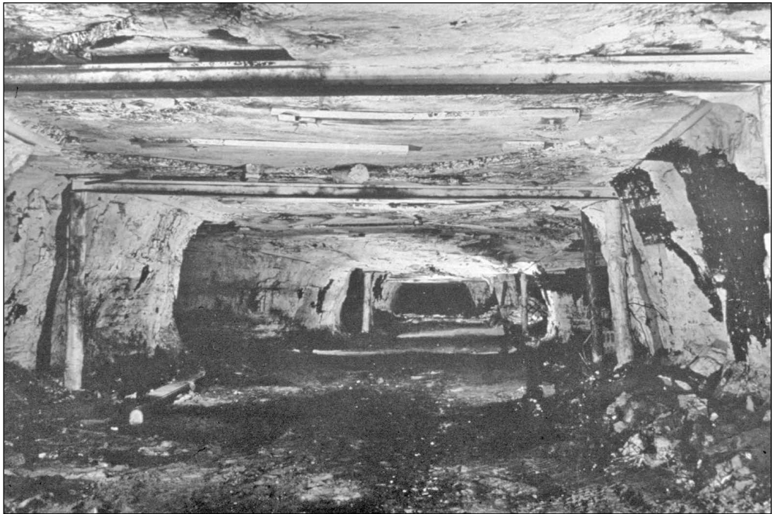
Figure 143 Peabody Coal Company, No. 10 Mine, Christian County. Timbering, steel I-beam, and roof bolting combined to keep this entry and haulage route open. The pillar outlines are characteristic of those used for conventional mining, where the coal is undercut and then shot down with permissible explosives (Ledvina et al. 1992). The white appearance of the pillars and roof is caused by rock dust.
