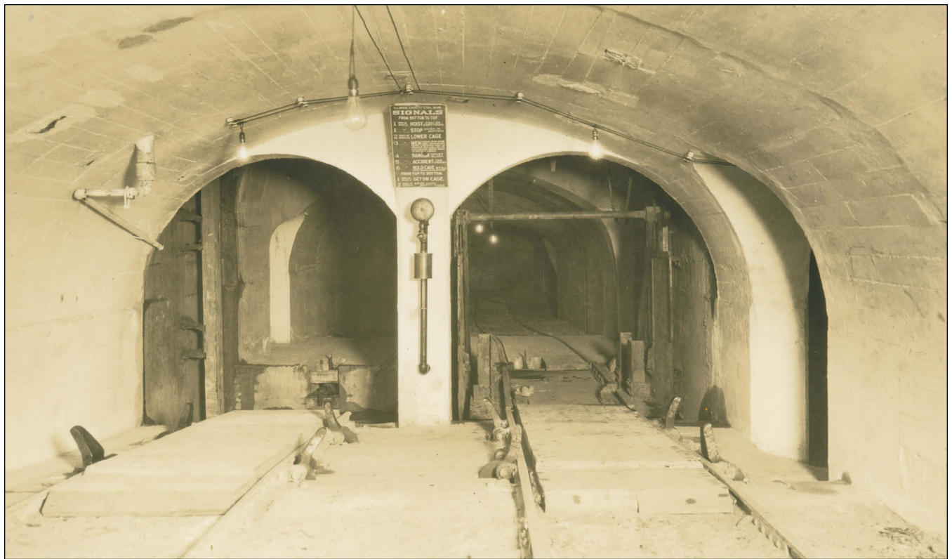
Figure 113 Big Creek Coals, Inc., No. 4 Mine, Saline County. This shaft bottom is 500 feet below the surface and is constructed of concrete. Mine cars loaded with coal are automatically caged and hoisted; the coal is emptied in 30 seconds. The round trip for each car is 3 minutes (Ledvina et al. 1992). The sign translating the signals is shown in detail on the following page.
