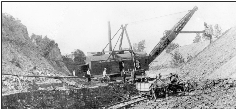
Figure 176 Mission Mining Company, Missionfield Mine, Vermilion County. The Marion Model 250 is shown removing overburden west of Danville.
