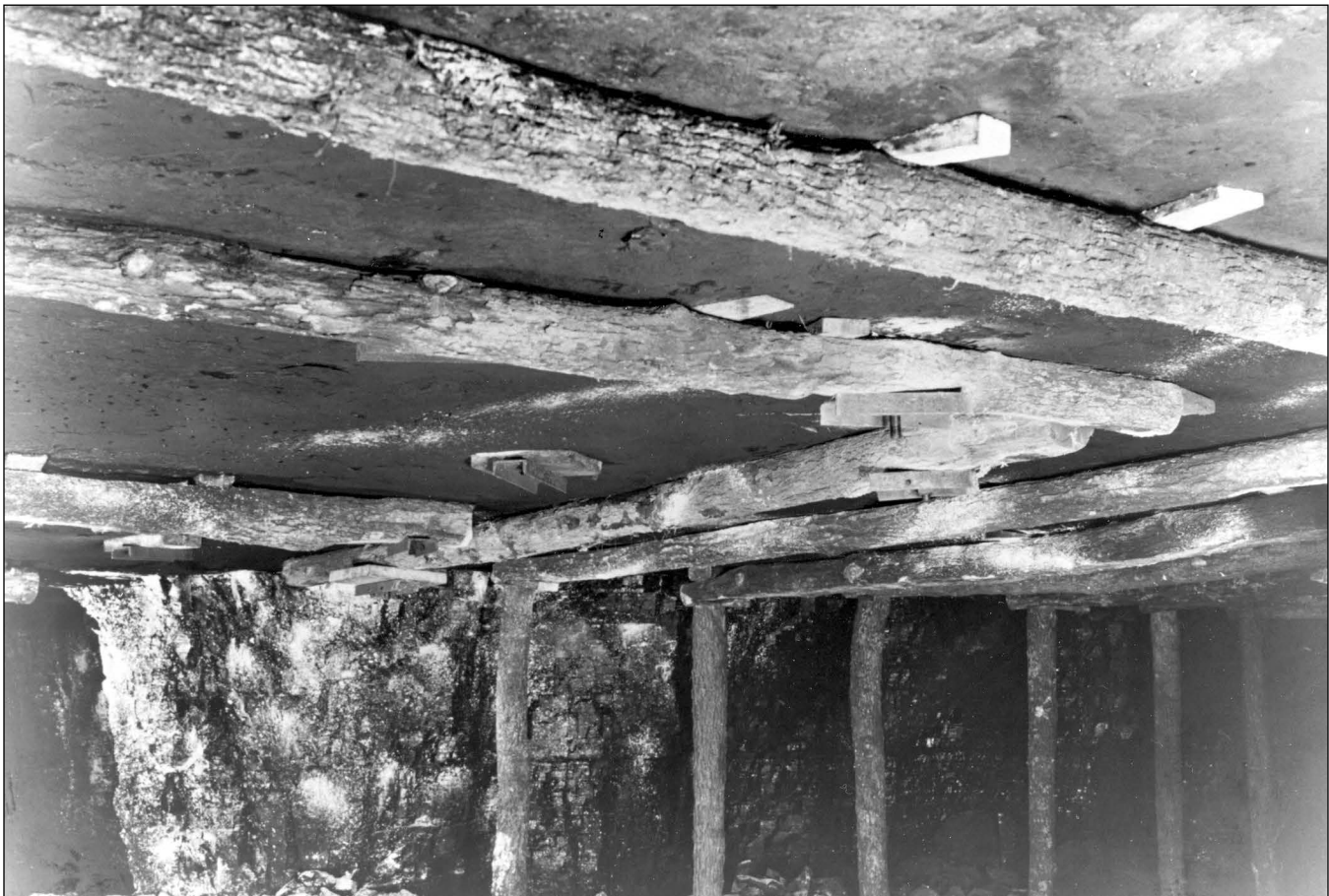
Courtesy Consolidated Coal Company | 1946
