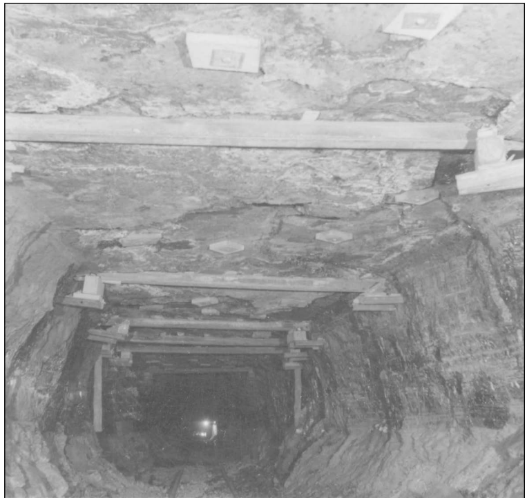
Figure 153 Freeman Coal Company, Crown Mine, Montgomery County. Near the coal hoist bottom, the combined use of bolts and steel bar supports can be seen.
