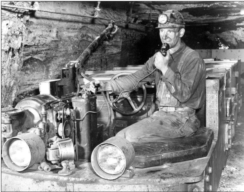
Figure 70 Bell & Zoller Coal Company, No. 2 Mine, near Zeigler, Franklin County. Trolley phones used a high-frequency carrier to conduct a signal through the trolley wire, thus providing communication throughout the mine. Here the motorman is speaking to the dispatcher from a 15-ton locomotive (Ledvina et al. 1992).
