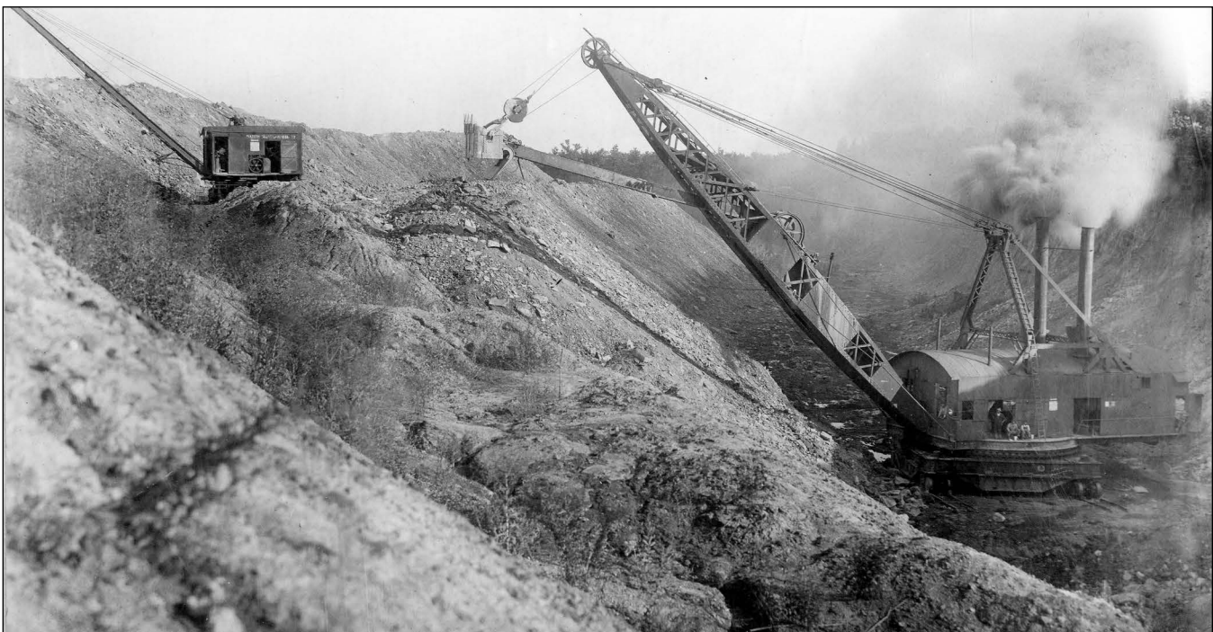
Figure 195 Mine unknown, probably in Vermilion County. A large rail-mounted steam shovel transfers spoil up the highwall. A smaller machine up on the spoil pile, a small crawler-mounted Marion Model 37 dragline, moves that spoil further away in a continuing effort to access deeper coal.
