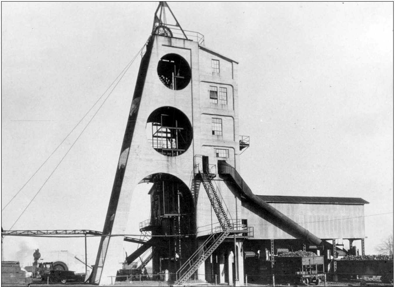
Figure 7 Sahara Coal Company, No. 1 Mine, Saline County. This reinforced concrete head frame was unusual; most were constructed of wood or metal.
