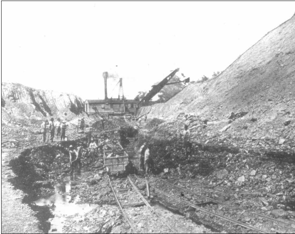
Figure 180 Danville area, Vermillion County. Hand loading was preferable in some mines even when small steam shovels were available. Some coal seams have two or more benches separated by bands of shale, and it was more efficient to leave that shale in the pit. Hand loading of the coals could contribute to the cleaning process by saving time and labor in the sorting sheds.
