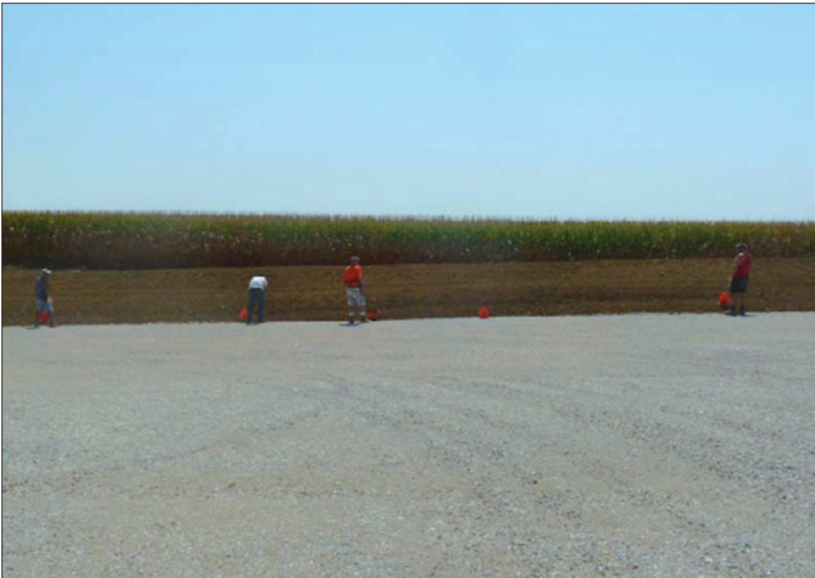
Figure D2 Taking a reading at 20-foot a-spacing, where the interval between electrodes is 20 feet, along south edge of the gravel pad. The 2-outer reels are the current electrodes and the inner ones are potential.
