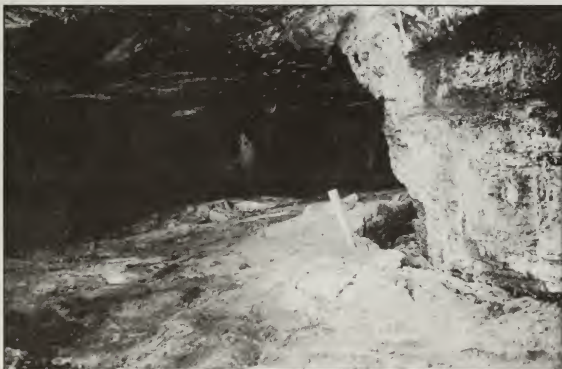
Figure 19 Floor squeeze in an underground mine in the Herrin Coal, Zeigler No. 5 Mine, Douglas County (Coal Section files, ISGS).
