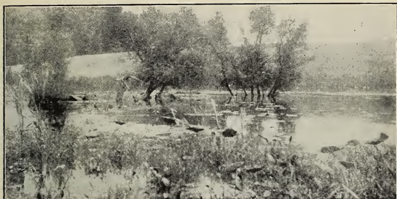
A. Upper reservoir of the Waterloo public water system.
