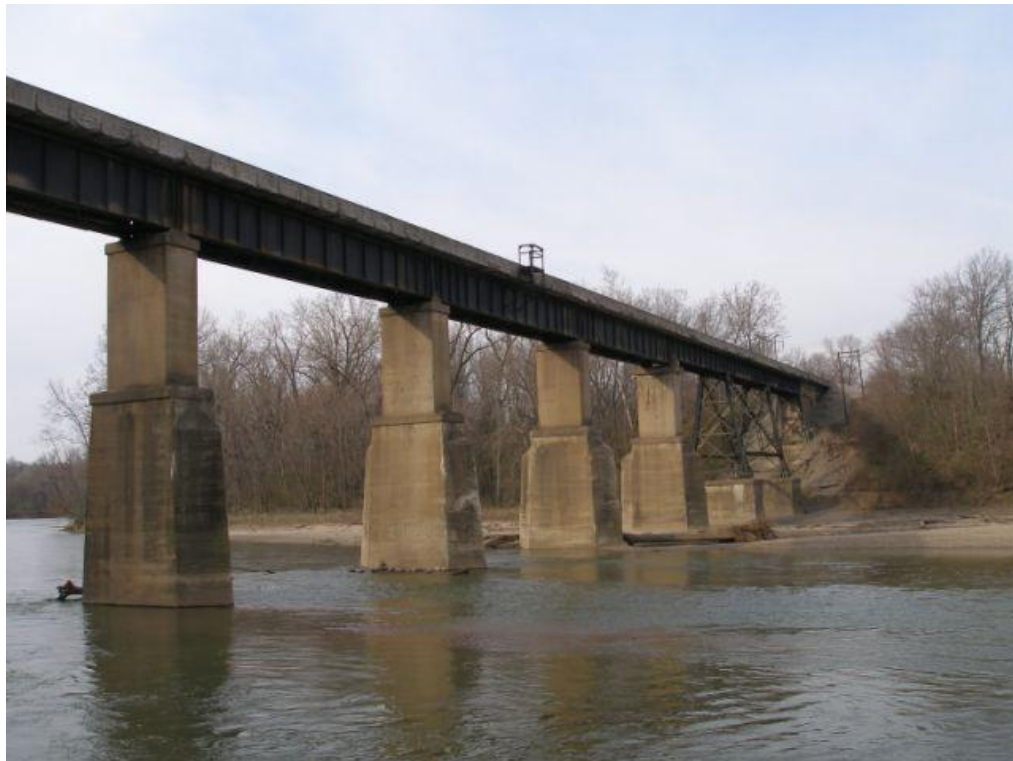
Figure 3.12. Vintage DPG used for HAL testing at FAST track at its original location (Photo Courtesy of TTCI (AAR)).
