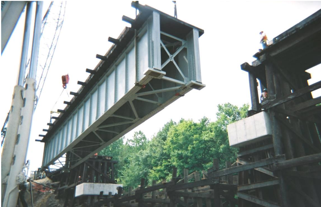
Figure 1.1. Railroad timber trestle bridge replacement, using a DPG member.
