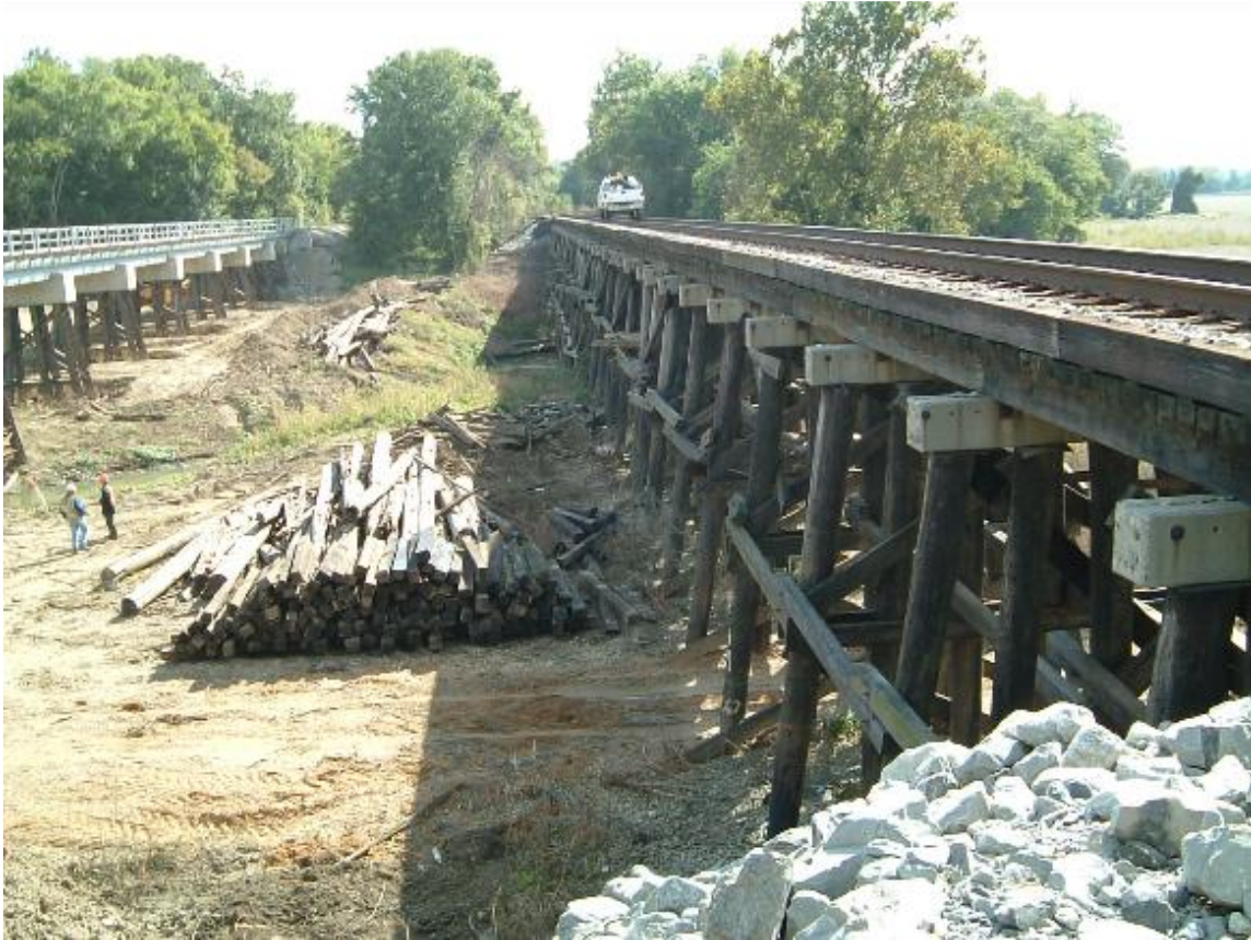
Figure 4.7. Wireless sensors installation in a timber trestle railroad bridge.
