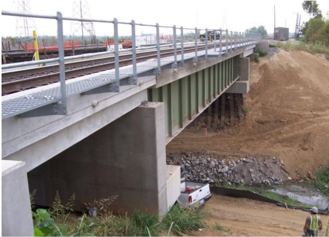
Figure 4.14. Typical new DPGs replacing an old railroad timber trestle (phase II).
