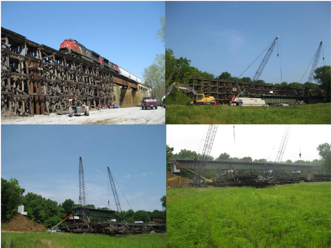
Figure 2.1. Railroad bridge trestle replacement using several DPGs in North America.
