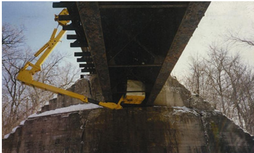
Figure 4.5. Railroad bridge inspection conducted from the railroad track (Sweeney and Unsworth, 2008).
