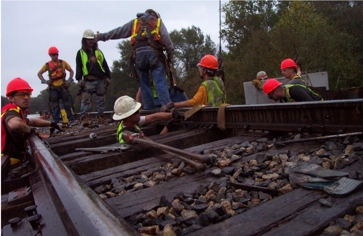
Figure 5.3. Backwall installation for a work window between trains.
