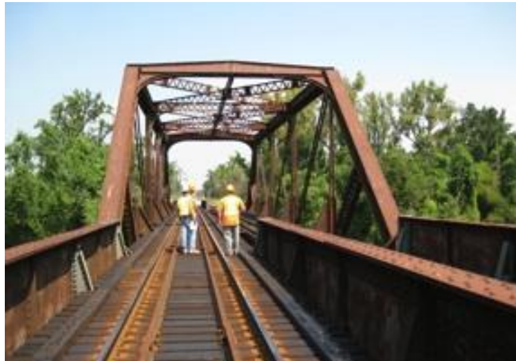
Figure 6.6. Railroad bridge inspection looking for local damage.
