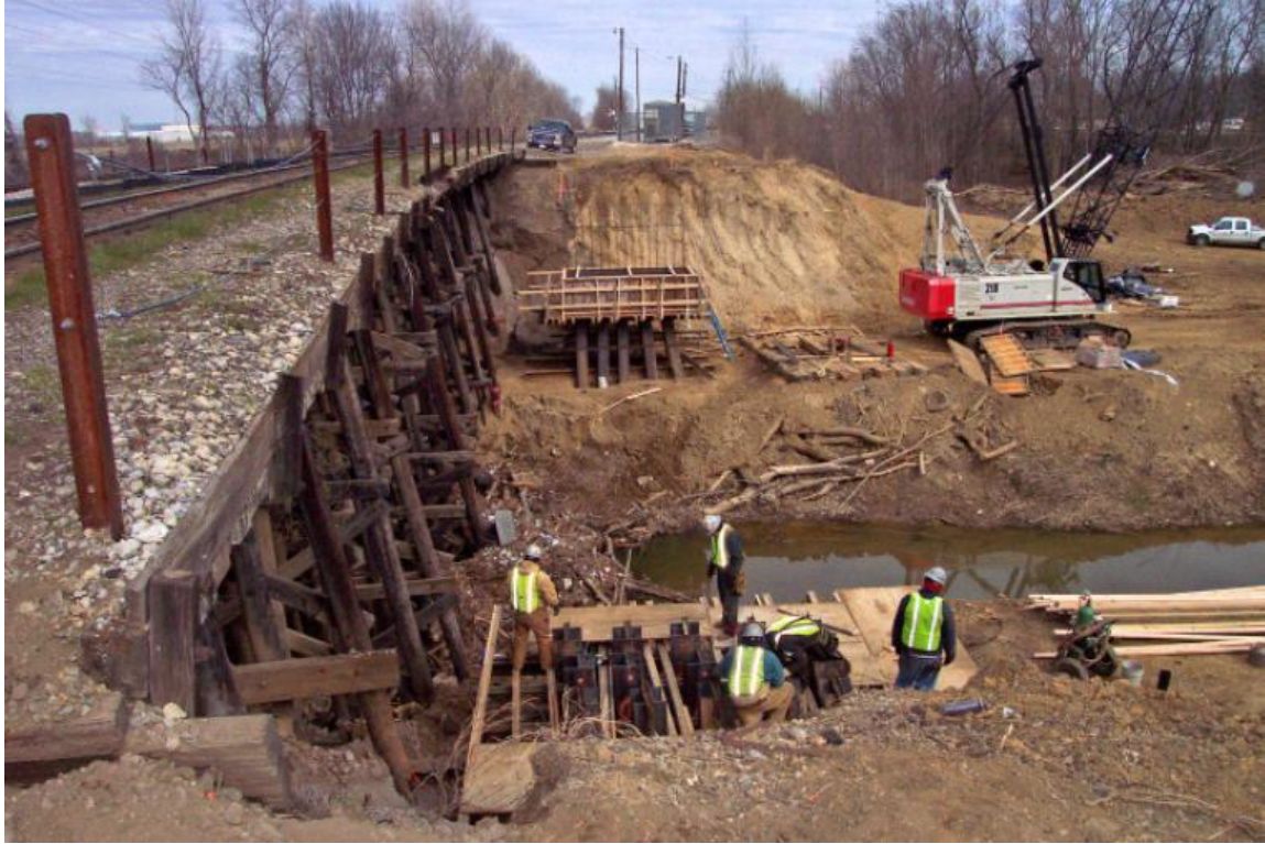
Figure 4.13. Typical timber trestle upgrade by DPGs on concrete abutments (phase I).
