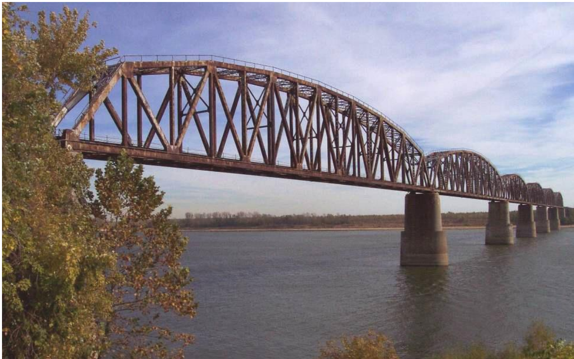
Figure 3.4. Cairo bridge over the Ohio river between Illinois and Kentucky.
