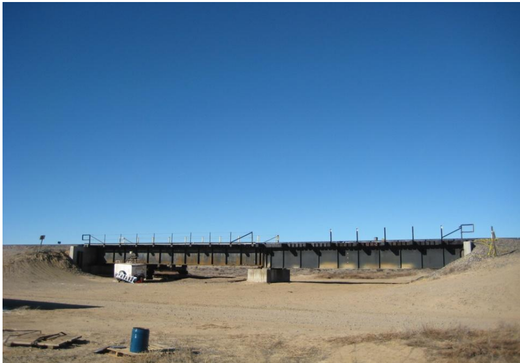
Figure 3.13. DPG installed at Pueblo, Colorado FAST track (Photo Courtesy of TTCI (AAR)).
