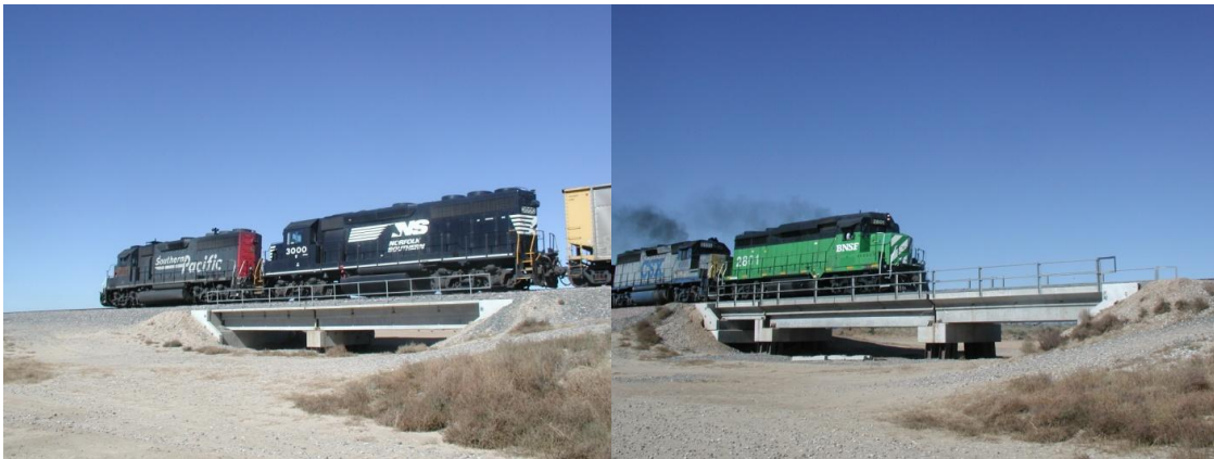
Figure 3.11. PC bridges under HAL testing at Pueblo, Colorado (Photo courtesy of TTCI (AAR)).
