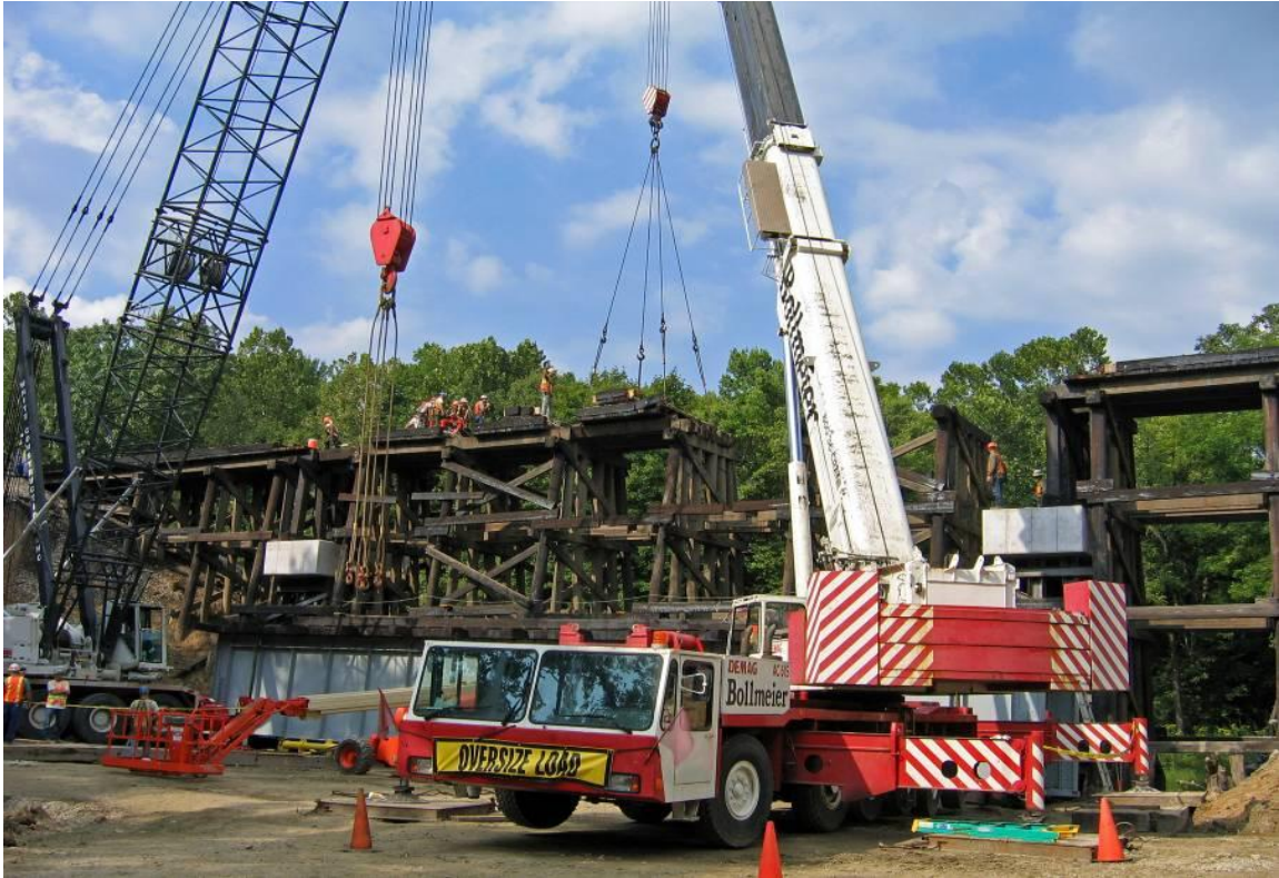
Figure 4.15. Timber trestle replacement in Cruse, Illinois.
