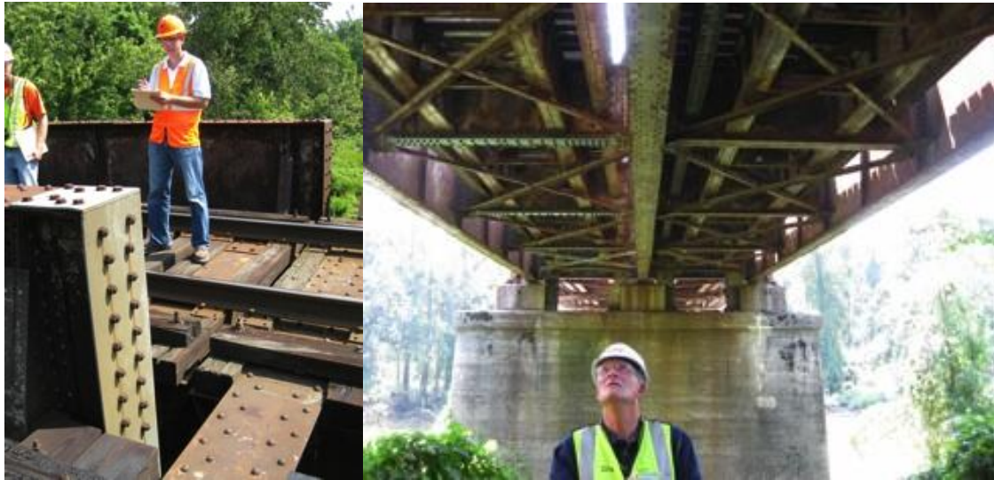
Figure 4.1. Bridge inspections for a Class I railroad TPGs from track level (left) and below track level (right).
