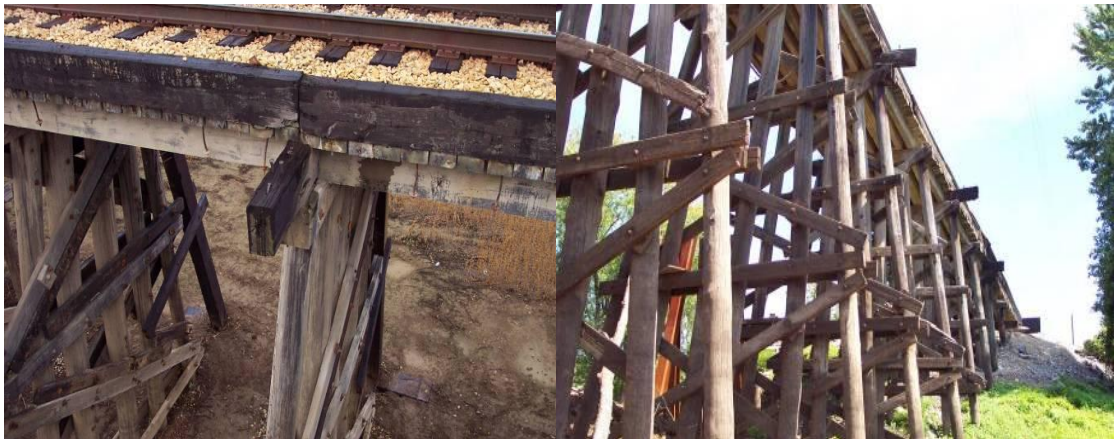
Figure 4.10. Timber trestle in use by a Class I railroad in Kentucky.
