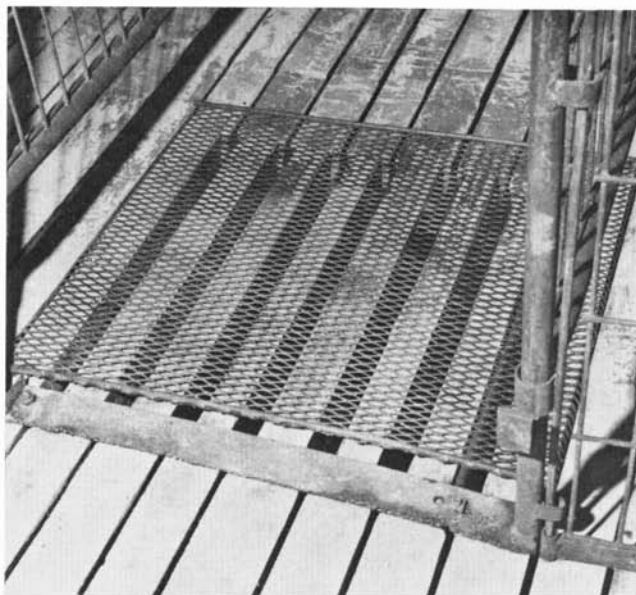
Fig. 21. Concrete slats with 1-inch spacing behind sow. Cover wide gaps during farrowing.
