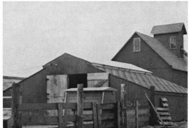
Fig. 4. Portable farrowing houses can be large enough for several sows. These multiple-unit portable farrowing houses are typical of many used in Illinois.
