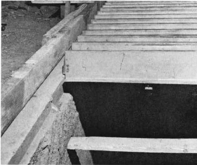
Fig. 19. Commercial cast-in-place metal forms for concrete slats.
