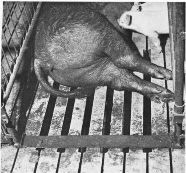
Fig. 21. Concrete slats with 1-inch spacing behind sow. Cover wide gaps during farrowing.
