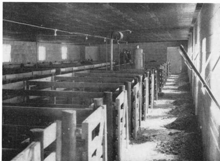
An insulated farrowing house equipped with exhaust fan and space heater. (Fig. 15)
