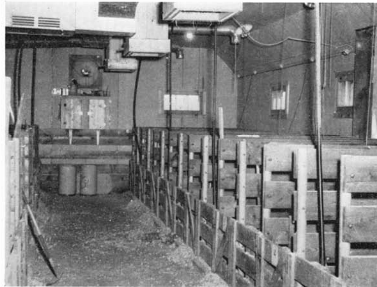
An insulated farrowing house equipped with exhaust fan and space heater. (Fig. 15)
