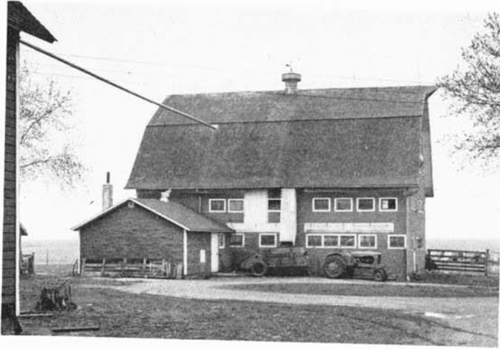
Converting a livestock barn with a sound structure into a multiple-story laying house is an economical use of a fixed investment.
