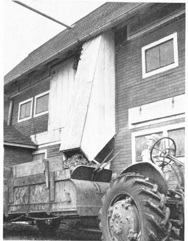
An enclosed manure chute on the side of a multiple-story house saves labor in loading the spreader. And it helps to keep the farmstead clean.
