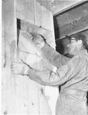
Cobs from freshly shelled corn are ground and blown into the top floor of this converted barn (left). Here they stay in good condition while serving as insulation for the lower floors. When litter material is needed, it can be dropped to the lower floors through a chute (right).
