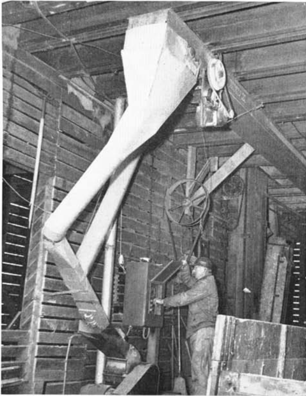
Grinding, mixing, and feeding are combined in a single operation with an electric blending mill, blowers, and mechanical feeders. Grain from overhead bins in the corn crib is mixed in the mill (above) into an all-mash ration, which is blown to the converted dairy barn where it flows directly into the mechanical feeders (right).
