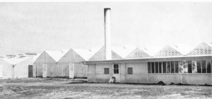
This large range of glass greenhouses is used for growing tomatoes. A headhouse with boiler room, storage, and work area connects the ends of the greenhouses. (Fig. 2)
