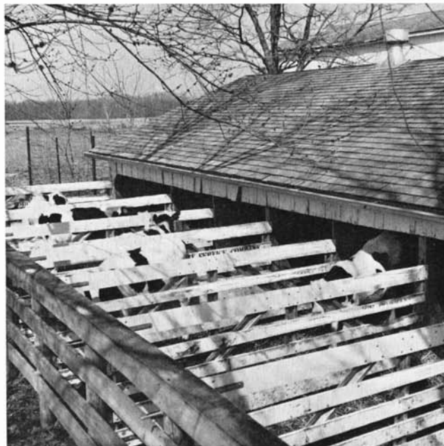
An existing building that has been converted to a good open-front calf barn. (Fig. 10)
