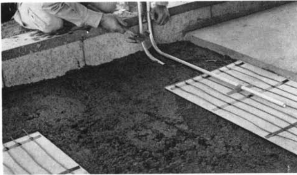
Installing conduit to protect wires and capillary tubes. (Fig. 13)
