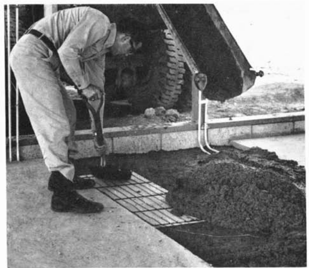
Covering heating unit with concrete.
