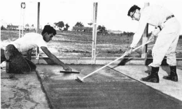
Finishing the concrete floor. (Fig. 16)
