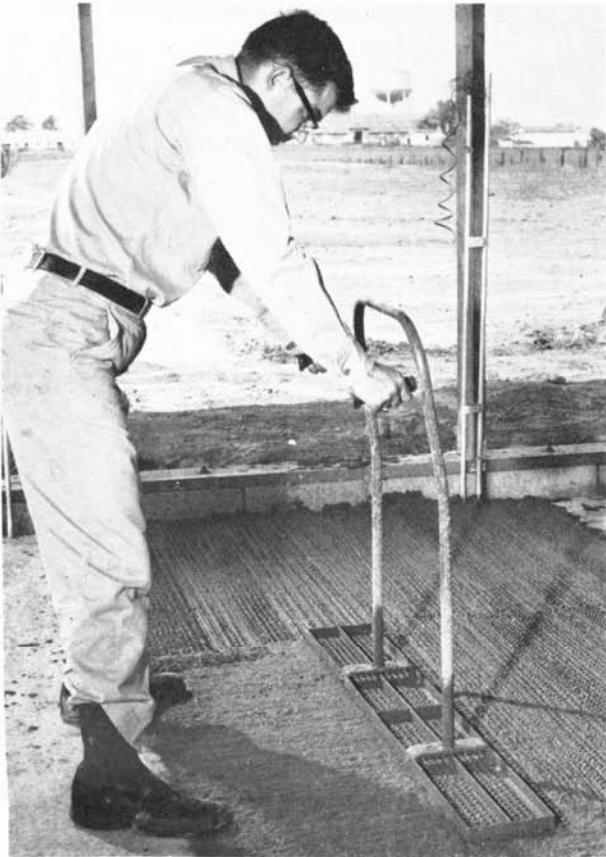
Tamping the concrete with a "jitterbug." (Fig. 15)
