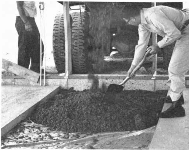
Carefully placing concrete over the vapor barrier.
