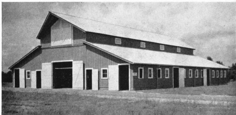
A popular type of cattle barn. The middle section holds hay resting on the ground. Cattle are fed on the sides from racks surrounding the hay. (Fig. 8)
