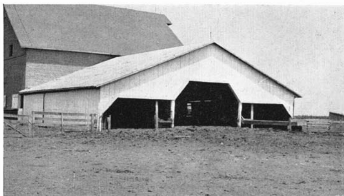
A cheap and satisfactory open-front cattle shelter. This 40-by-50-foot building shelters about 100 weanling steers until they are fat a year later. (Fig. 10)
