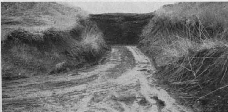
Good drainage and a paved floor are essential for a trench silo. It is desirable to line the sidewalls, but earth sidewalls can be used if they have enough slope to prevent crumbling. This trench has a good floor and drainage, but the sidewalls should have been given more slope.
