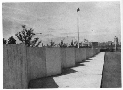
The illustration above shows a unique method for screening a parking area, achieved by using a stepped diagonal concrete wall. Notice the interesting shadow pattern cast by the wall on the pedestrian walk located at the edge of the parking lot.
