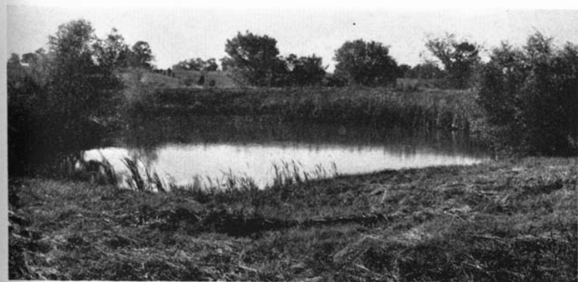
Farm ponds help solve the water problem on pasture. This pond was made by building an embankment across a gully. It has a 40-acre watershed.
