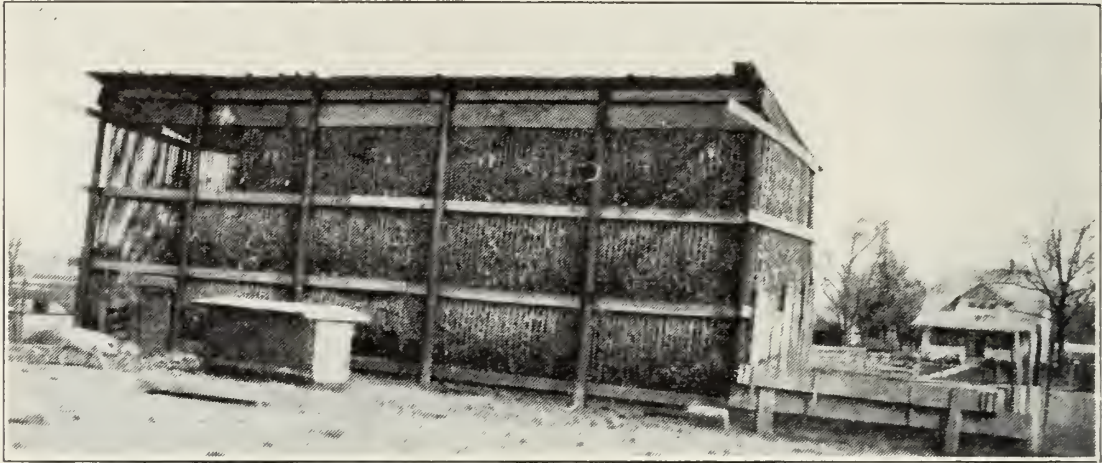
FIG. 10.—AN ECONOMICAL STORAGE OF CORN NEEDED FOR FEEDING
