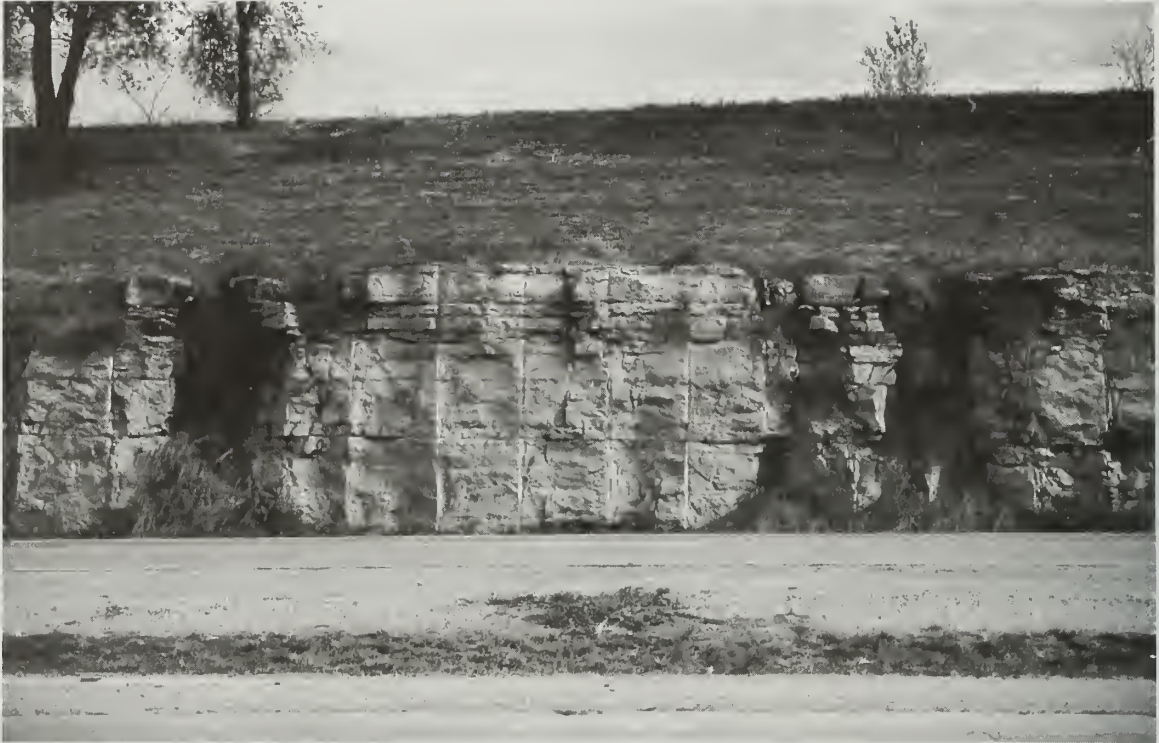
Figure 35 View of the contact between the top of the bedrock (Salem Limestone) and the overlying Quaternary sediments. Water percolating through the soil becomes more acidic and dissolves the limestone along joints. The joints have been enlarged by dissolution to the point where some of the rock has slid downward into the bedrock cavities. If the excavation for the highway had not taken place, this process would have continued and a small sinkhole likely would have formed. The darker surfaces of the rock are natural and show the effects of acidic groundwater etching, whereas the lighter surfaces are manmade and are the result of the excavation.
