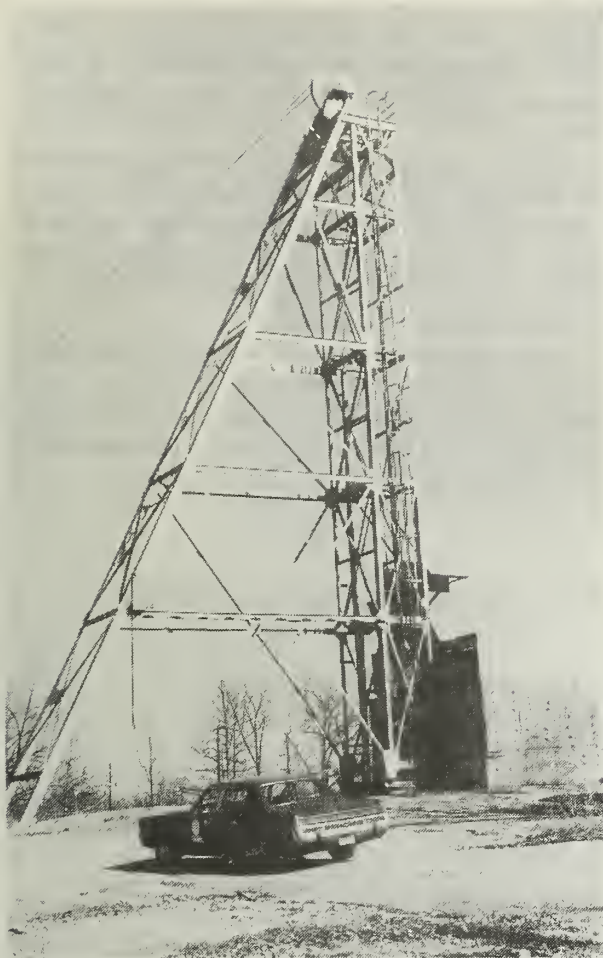
Figure KY-24. Tabb No. 1 shaft of Lafayette mine (inactive). This has been the main opening on the Tabb fault system.
