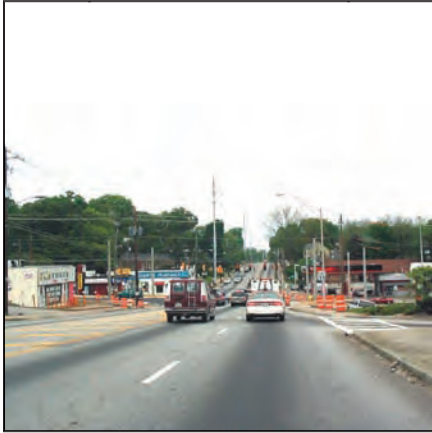
Moreland Avenue just north of I-20
