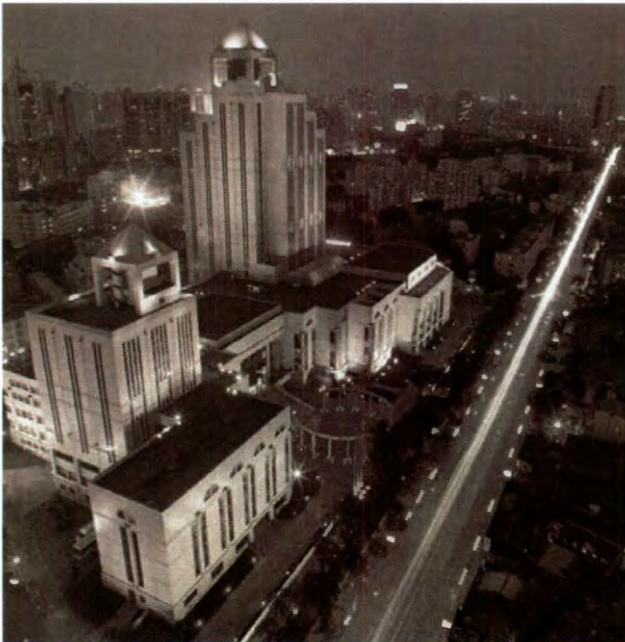
the institution of the public library provides a programmatic vehicle for extending the public realm onto a facade
