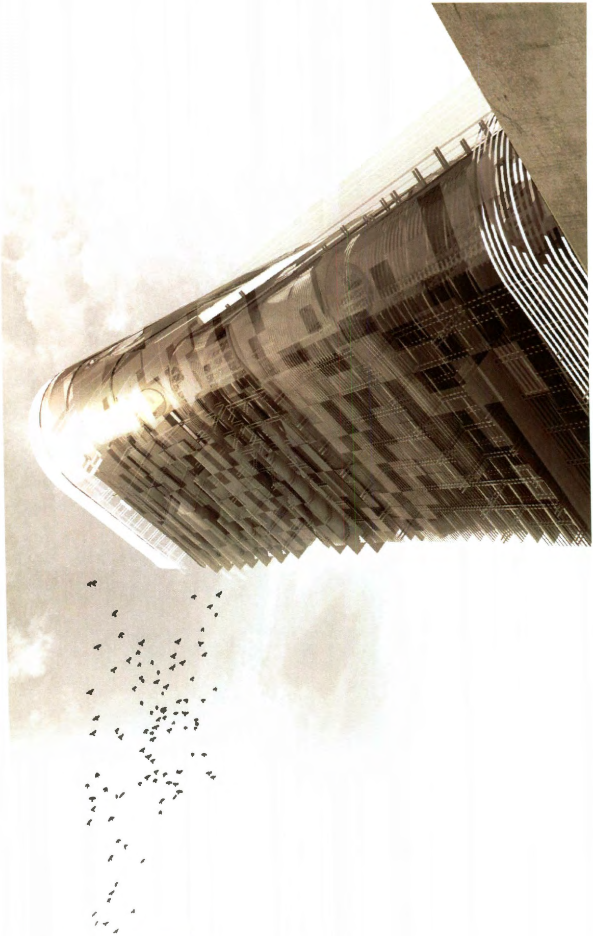
VIEW OF TOWER FROM BELOW
