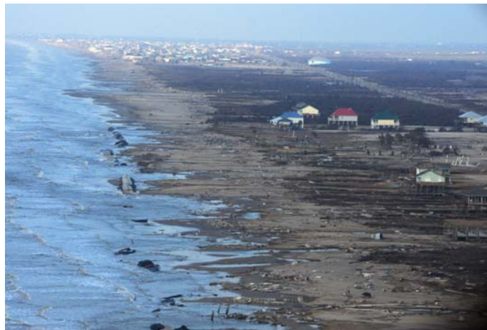
Figure 2-3: Bolivar Peninsula after Hurricane Ike made landfall on the Texas Coast (FEMA, 2008)
