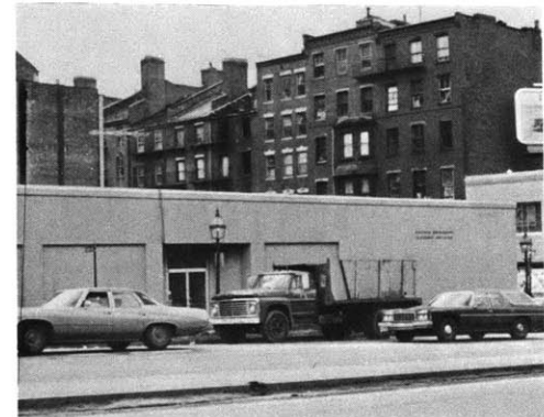
Suffolk's existing Ridgeway Building Cambridge Street facade
