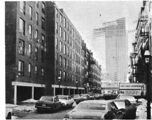
Fulton Street frontage
