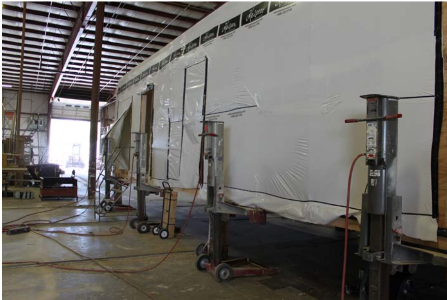
Figure 8 - Module ready to be set on trailer
