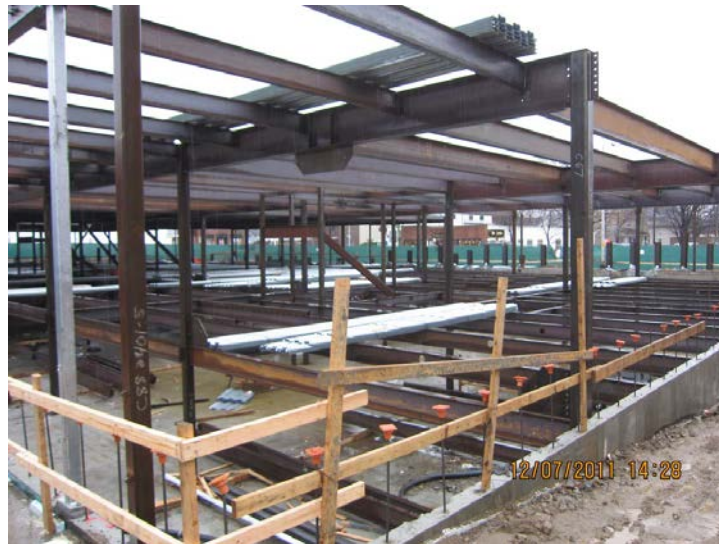
Figure 3 - Erecting the steel for the retail ground floor
