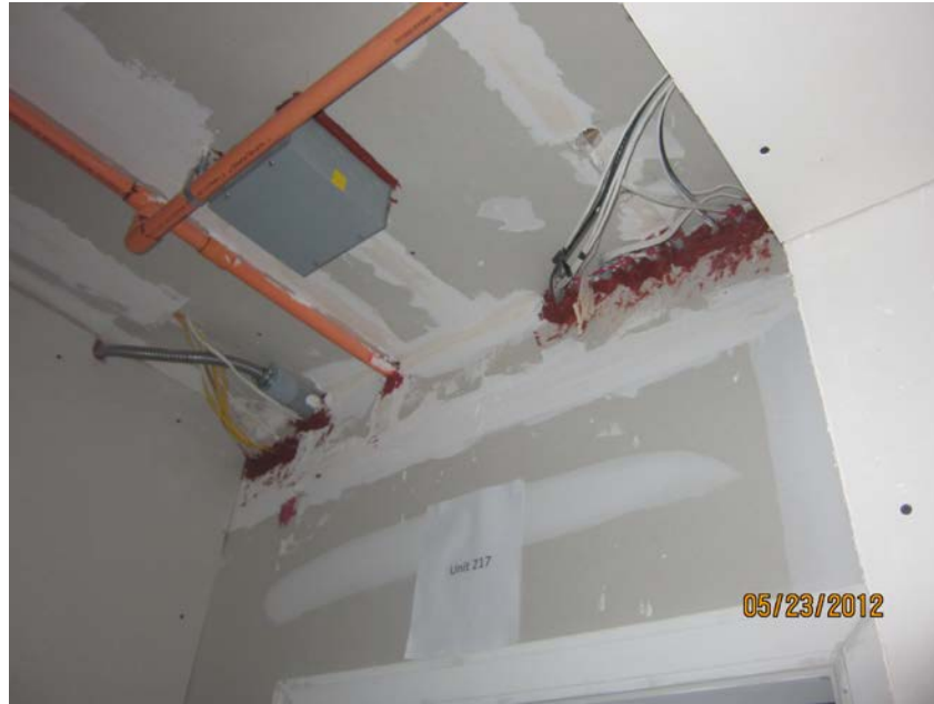
Figure 13 – Inside finishes and residual work on MEP connections
