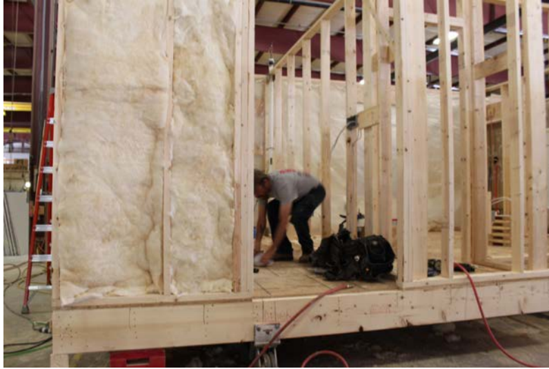
Figure 6 - Modules insulated and connections are made
