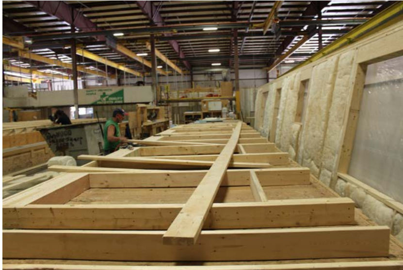
Figure 4 - Mill work modular pieces
