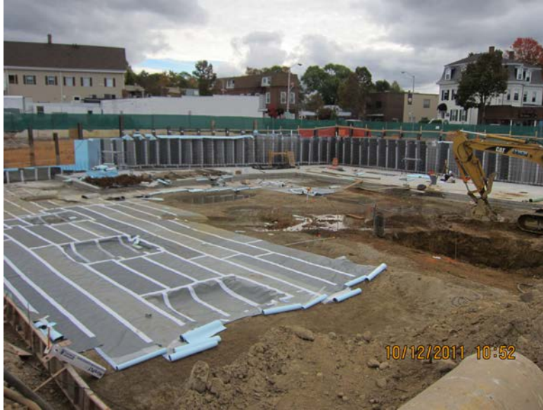
Figure 2 - Excavation and preparation for the foundation and underground parking
