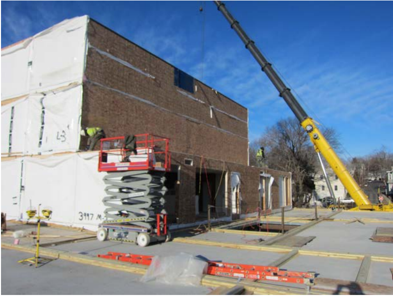
Figure 9 - A crane onsite stacks the modules together
