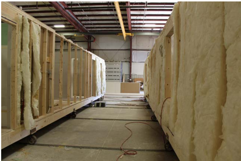
Figure 5 - Modules are framed and set on the tracks
