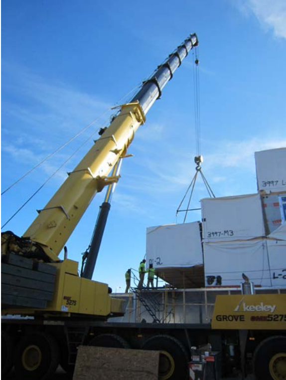
Figure 10 - A crane on site stacks the modules together (2)
