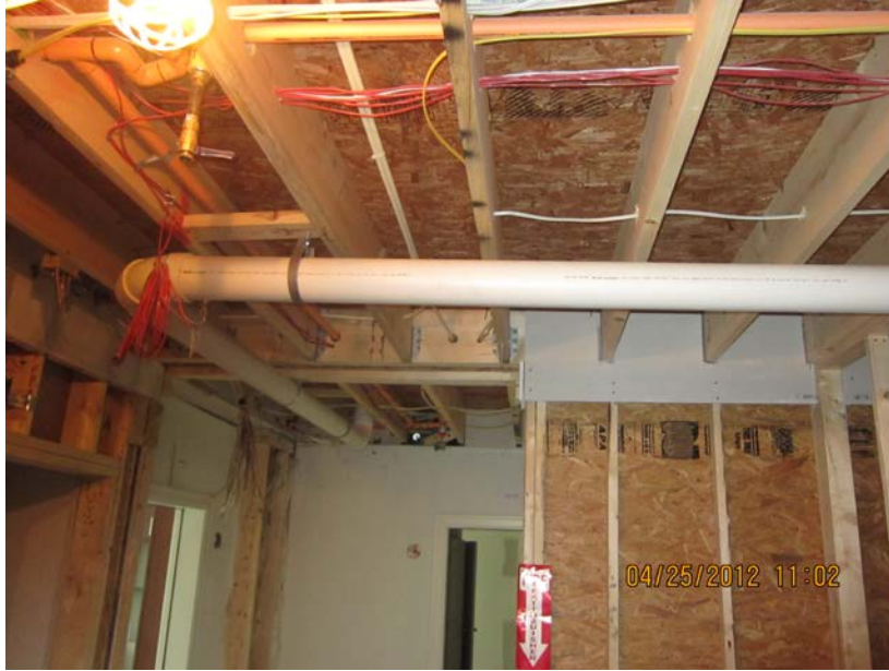
Figure 11 - Modules are set together and MEP systems are connected
