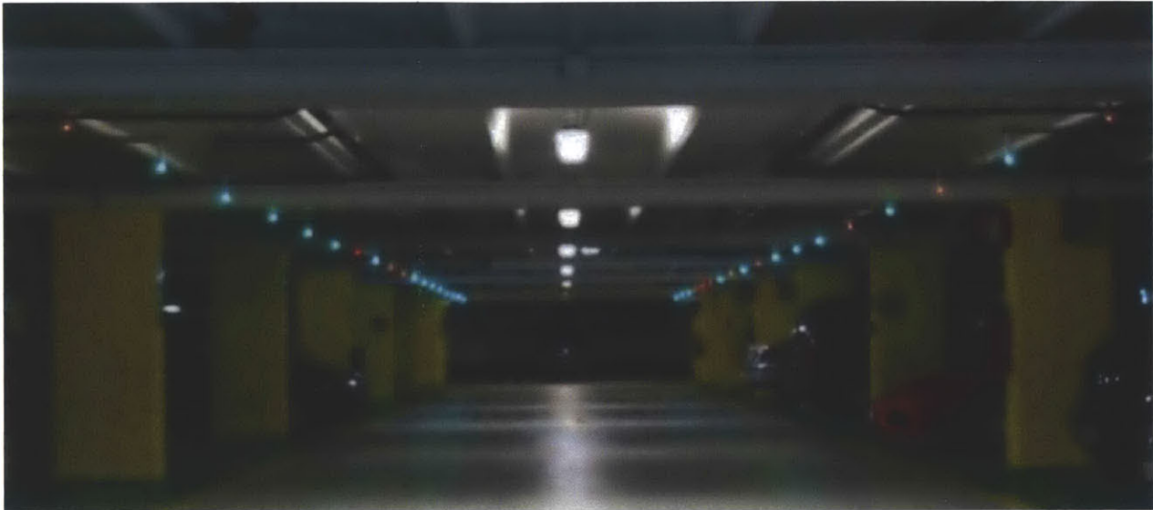
Figure 9: LED-based ambient information systems in parking garages provide real-time feedback to users about which parking spots are available. Green LEDs indicate available spots while red indicates occupied.
