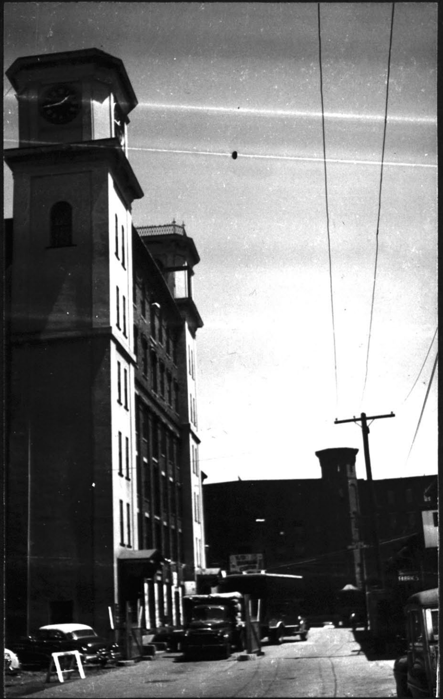
MILLS AT LOWELL, MASS. (RENOVATED)
