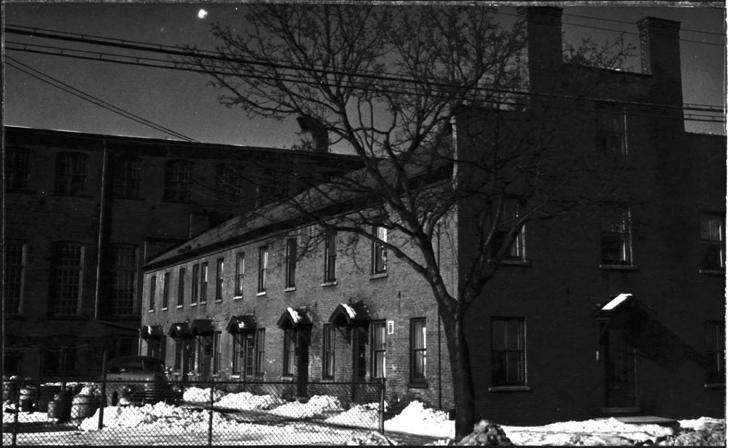
INDUSTRIAL HOUSING UNITS. L.L. BROWN PAPER CO. 1825 ADAMS.
