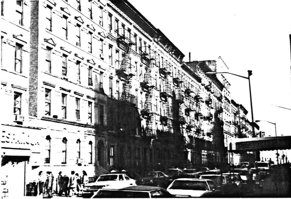
South side of the site on 109th St. at present.
