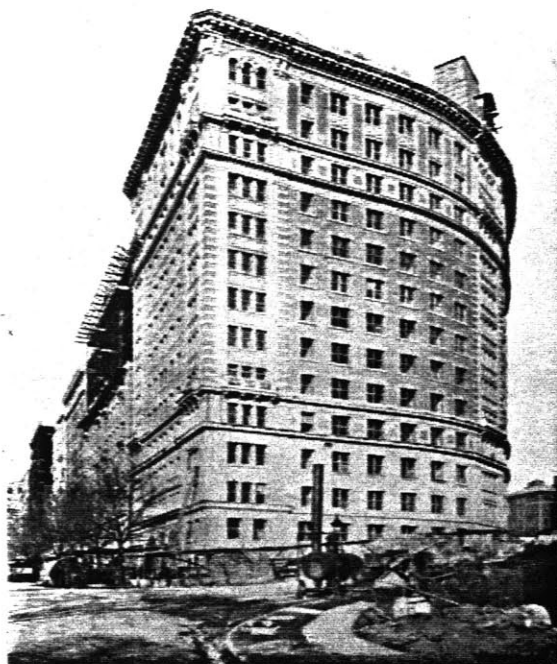
Riverside Drive under construction at 116th St., 1908.
