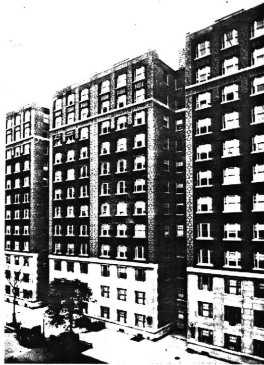
The Prince Humbert and the Marc Antony (Schwartz and Gross, 1910). These buildings are part of the continuous line of 150 ft. apartment houses on the south side of Cathedral Parkway.
