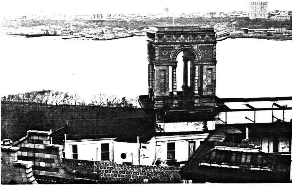
Ornamental cupola on the roof of the Hendrik Hudson, with Riverside Park and the Hudson River beyond.
