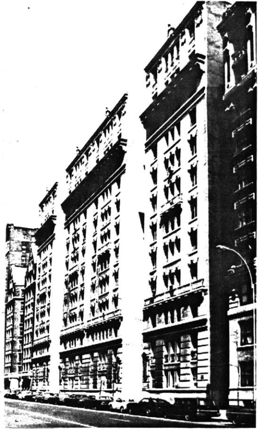
No. 509 Cathedral Parkway--somewhat unusual in having an all-limestone facade.
