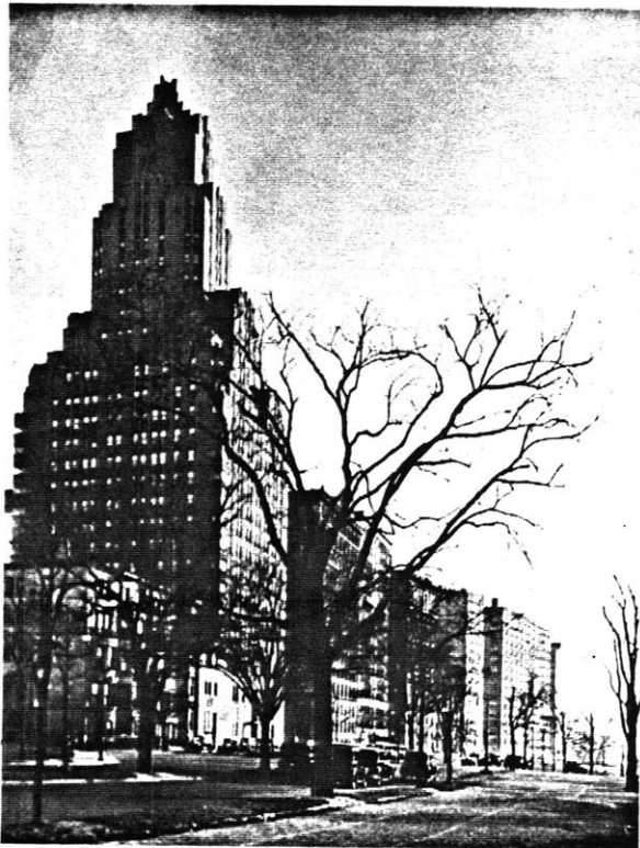
The Master Apartments and Roerich Museum, 103rd St. and Riverside Dr. (Helmle, Corbett & Harrison, 1929): View from the Drive shortly after its completion.
