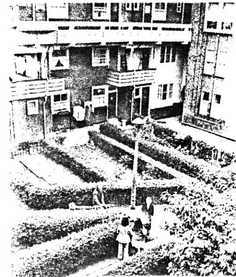
Public paths and private yards in Brinkman's Spangen, Rotter- dam.
