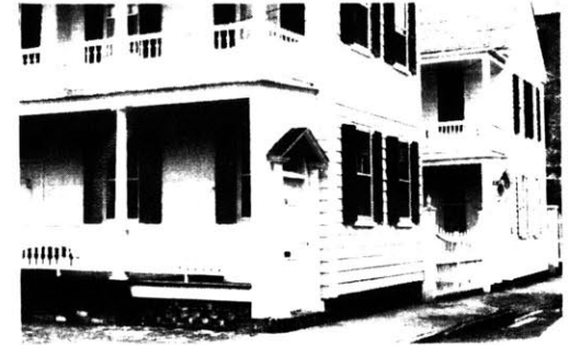
+ Housing perpendicular to street in Charlestown, S.C. All porches face South or East.
