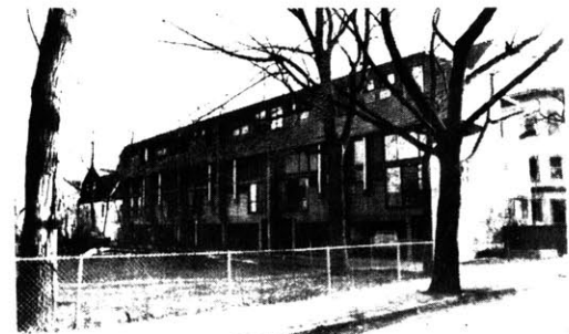
+ Problem: sideyards become a paved surface.
