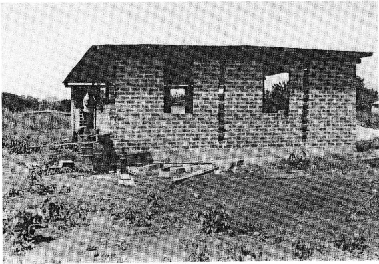
CONSTRUCTION OF INFILL WALLS
