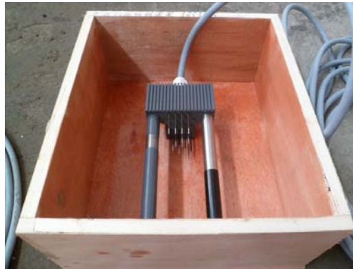
Fig-1: Sensor probe fixed in a wooden mould before pouring concrete
