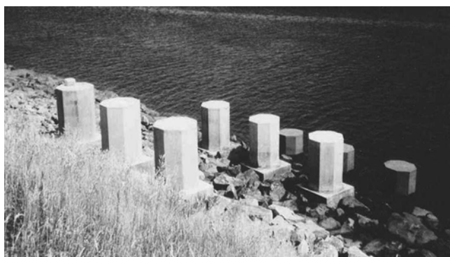
Fig. 1—Showing location of nine piers at marine exposure site; at this location, North Sea contains approximately 19.8 g/L (0.0436 lb/L) of chloride ions.
