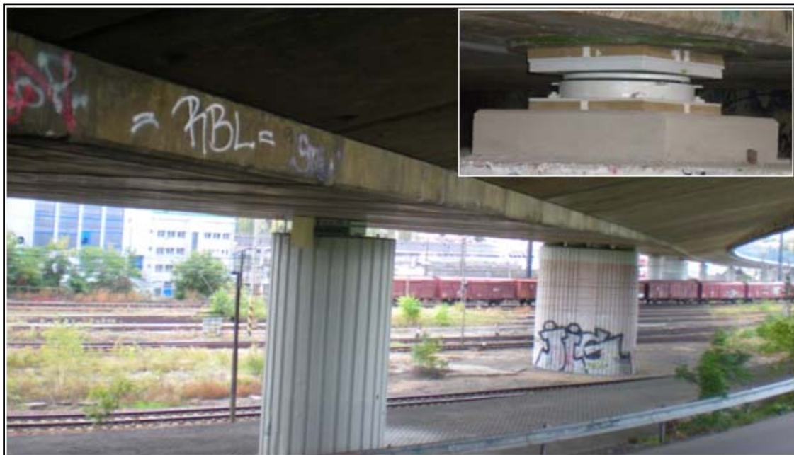
Fig. 22 - Simple and double bearings
