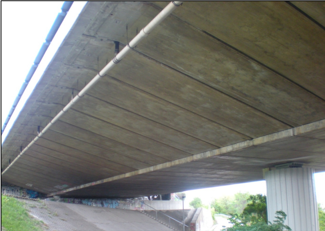
Fig. 13 - Particular of the concrete box section
