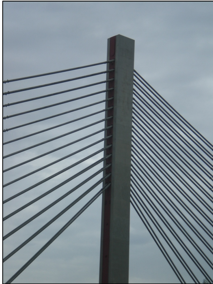
Fig. 17 - Top of the pylon
