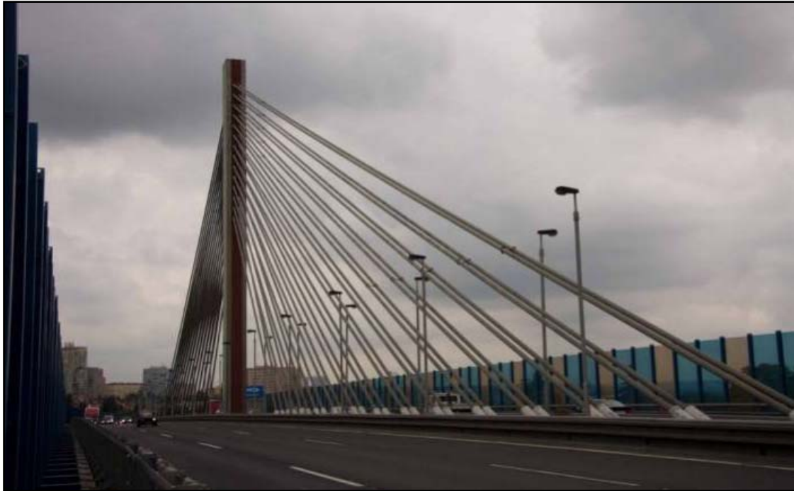
Fig. 21 - Cables connection to the deck
