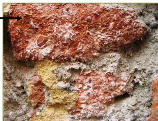
Figure 7: Example of masonry damaged due to the crystallization of salt on a frequent street in Prague, Czech Republic, where NaCl is used as a de-icing agent in winter
