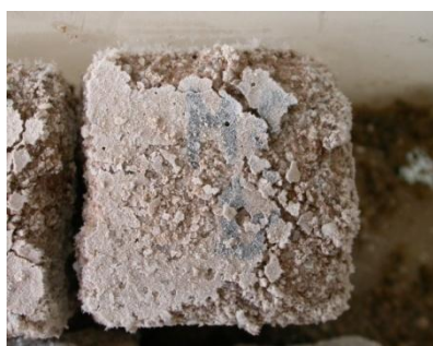
Figure 79: Surface scaling due to freeze-thaw cycling (sample BO 3 )
